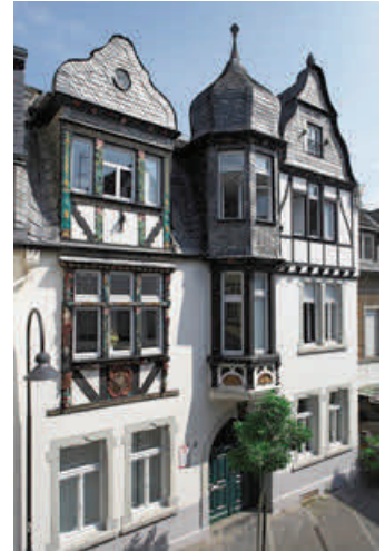
WHU Building Z: TIM-Chair Location
