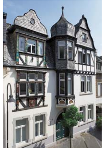
WHU Building Z: TIM-Chair Location
