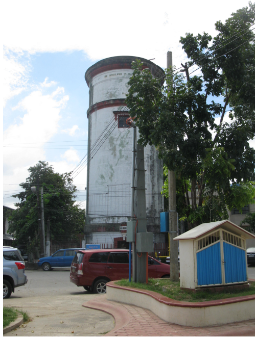
Figure 6. The Water Tower. Photo taken by the author, 2016.
