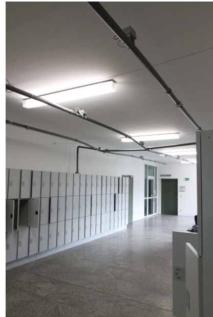
(d) Foyer: 20 sensors, 51 days, height 2.80m, and area 78m 2
