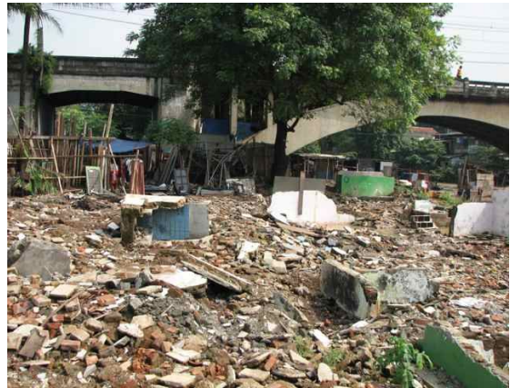
RW 10 RT 01 After its Demolition
