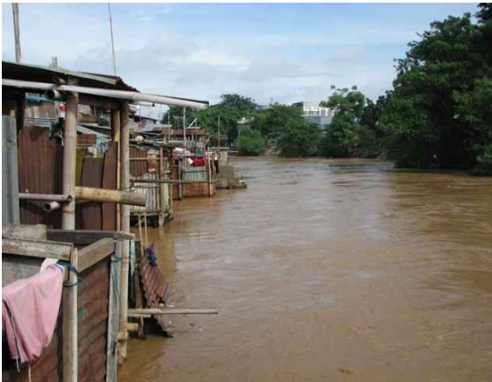
Public Toilets Built in Ciliwung River
