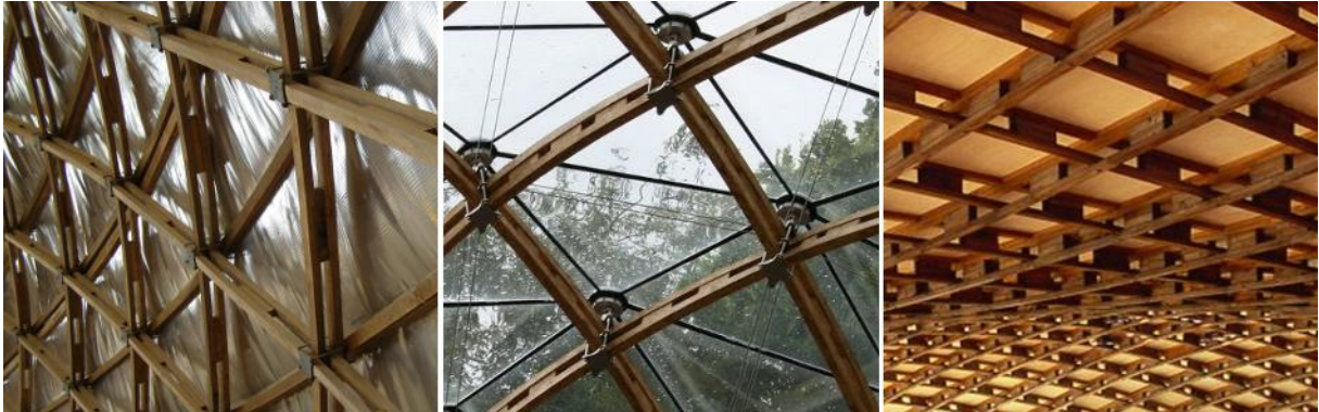
Figure 3-20: Different bracing elements on elastic gridshells
