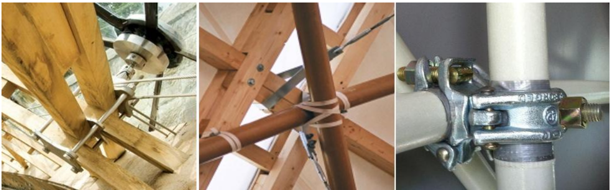
Figure 3-21: Different grid connections on elastic gridshells
