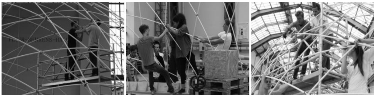
Figure 5-21: Assembling of bracing layer on the irregular hemisphere
