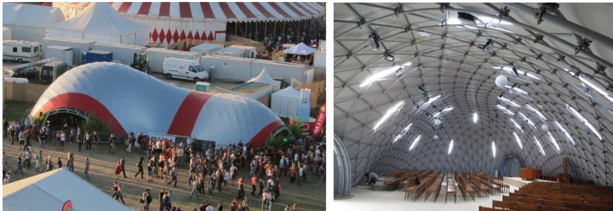
Figure 2-17: Examples of GFRP gridshells: Solidays' Festival (2011) at the left and Créteil Cathedral (2013) at the right
