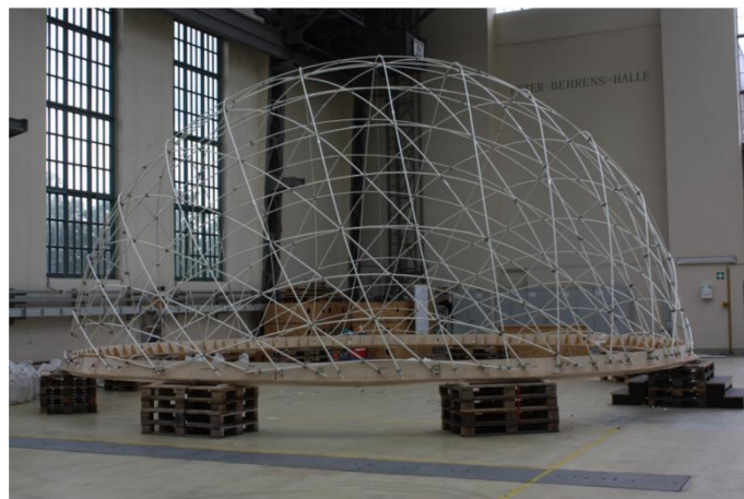
Figure 2-6: GFRP irregular gridshell with optimised curvature, Germany 2012
