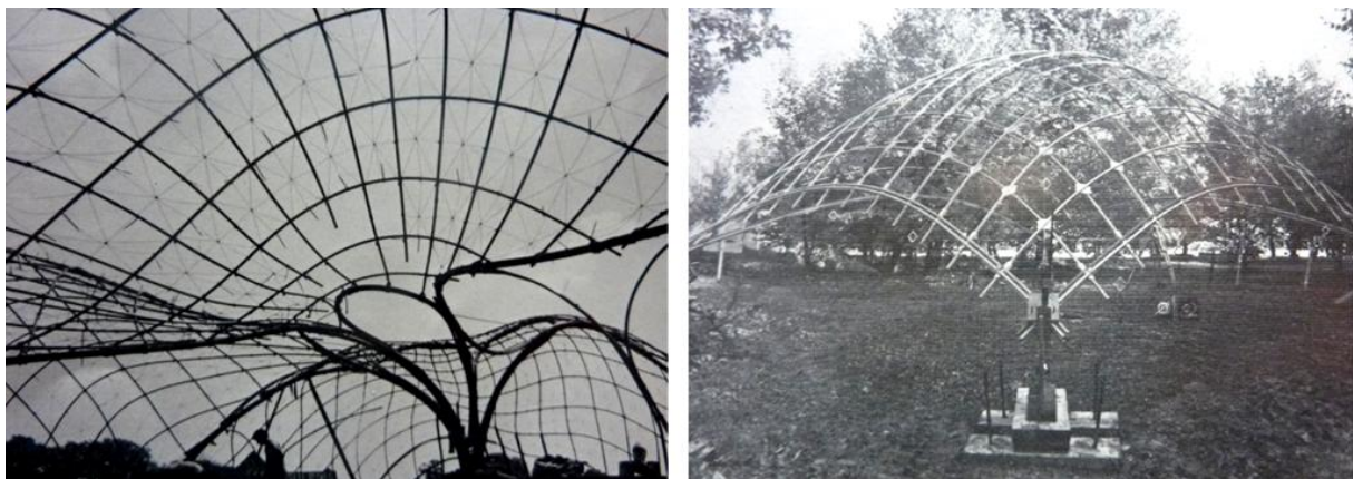
Figure 1-2: Research about bent geometry and structural behaviour of elastic gridshells with physical prototypes: (left) protective roof on a playground in Wandsworth Common executed by students of the North London Polytechnic in 1976 and (right) research structure constructed by students of the University of Stuttgart at the IL in 1976 [2]
