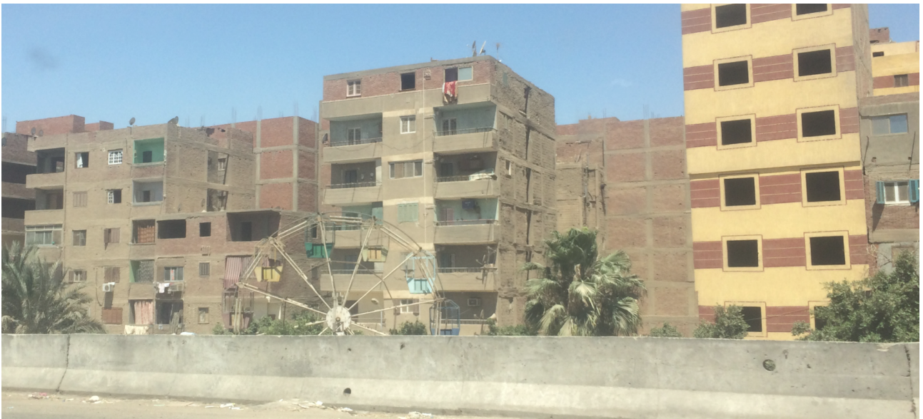
Figure 4.12.: Residential buildings in Giza (Abd El Latif Street on 25 April 2015).
