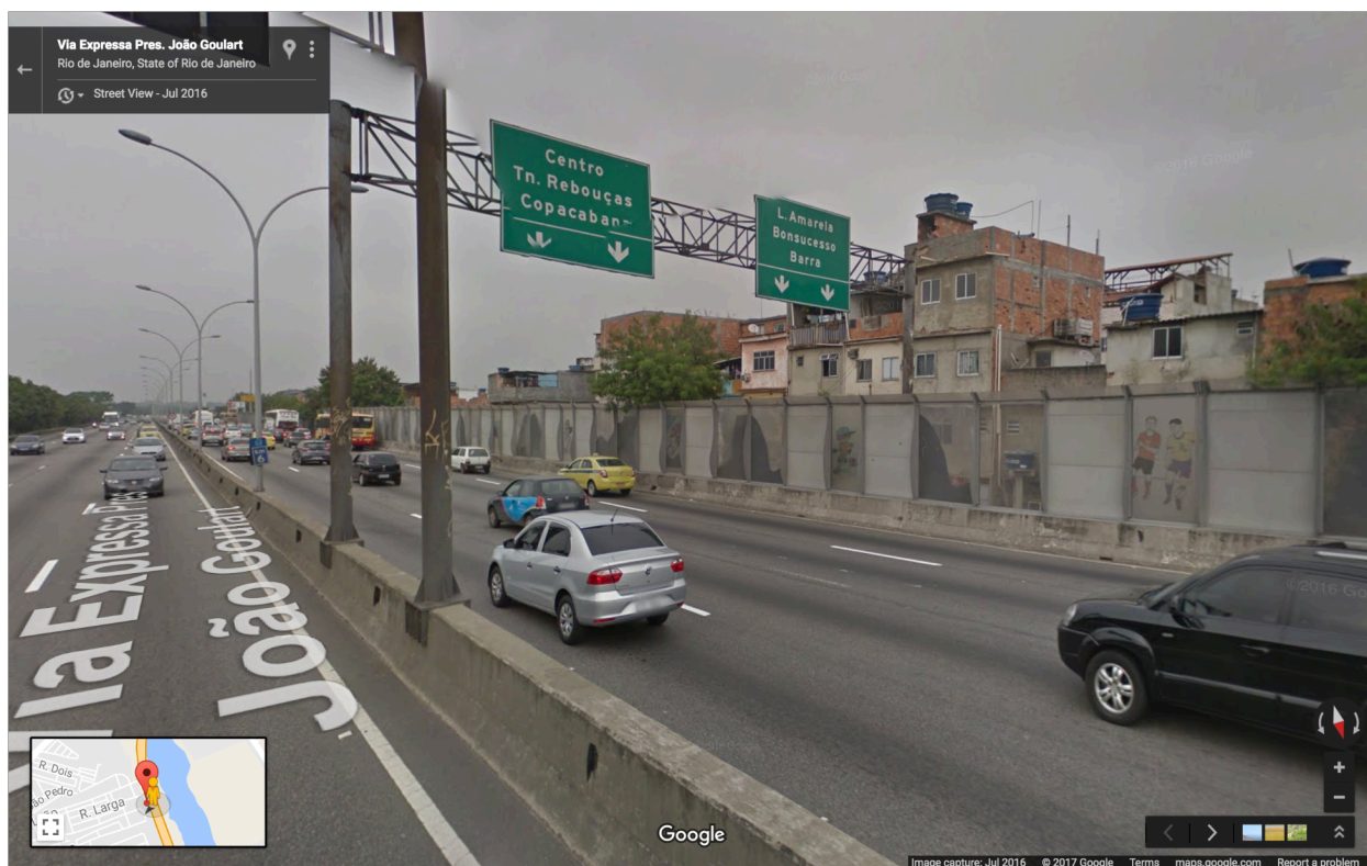
Fig. 35: General overview of the acoustic barrier of Maré .
