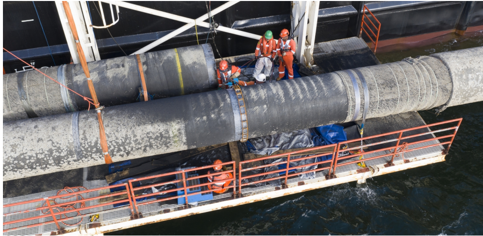
Figure 0.2.: Process of building the Nord Stream 2 pipeline 7 © Nord Stream 2, Axel Schmidt
