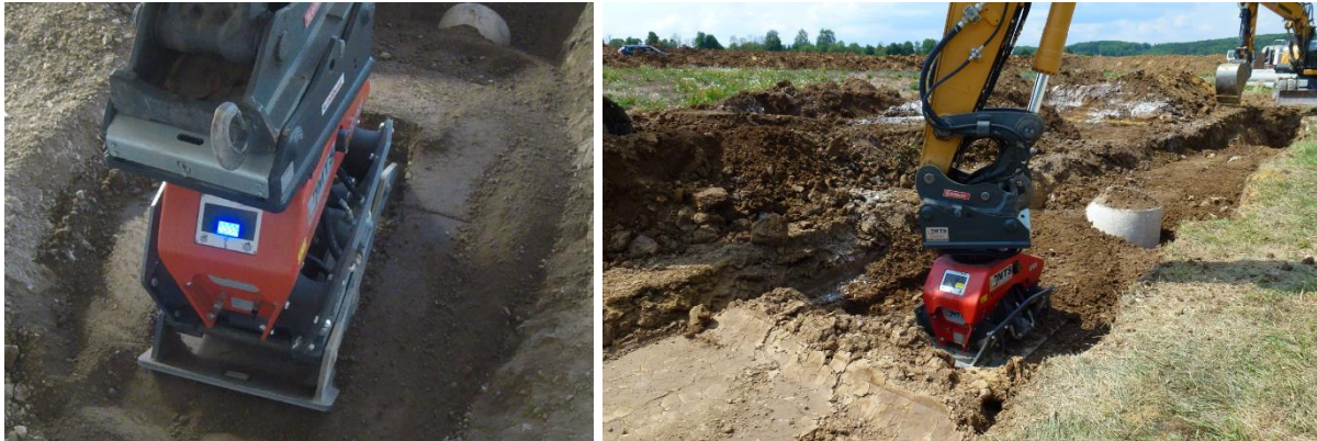
Figure 1: Attachment compactor compacting trench filling, with display screen
