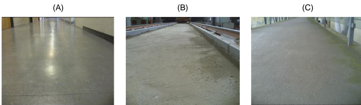
Figure 2: Three test areas: (A) linoleum, (B) compacted sand and (C) concrete.
