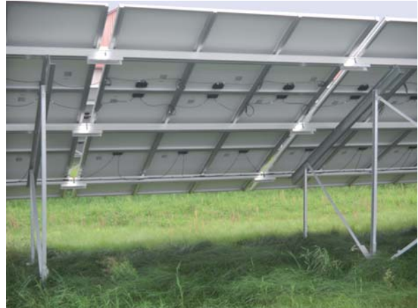
Figure 1: Example photovoltaic structure (case study a)
