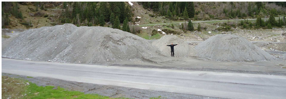
Figure 7.1.5: Sediment removed from the Fagge river delta and stored for further usage in construction (May 12, 2014). Master student Sebastian Wiggenhauser for scale reference.
