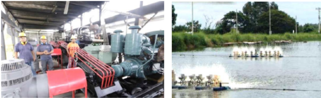
Figure 7. First electrified pumps (right) and aerators (left) in Ecuador Source: Cámara Nacional de Acuicultura (2017)
