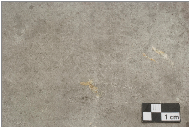
Abb. 225: Detail Filter 3 Detail, gelbliche Ablagerung
