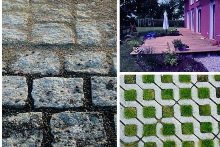
Figure 23 Permeable surface coverings are, for example, lawn grids (below right) or paving stone with chippings joints (left) in driveways, wooden gratings on terraces (top right). (Bayerisches Landesamt für Umwelt)
