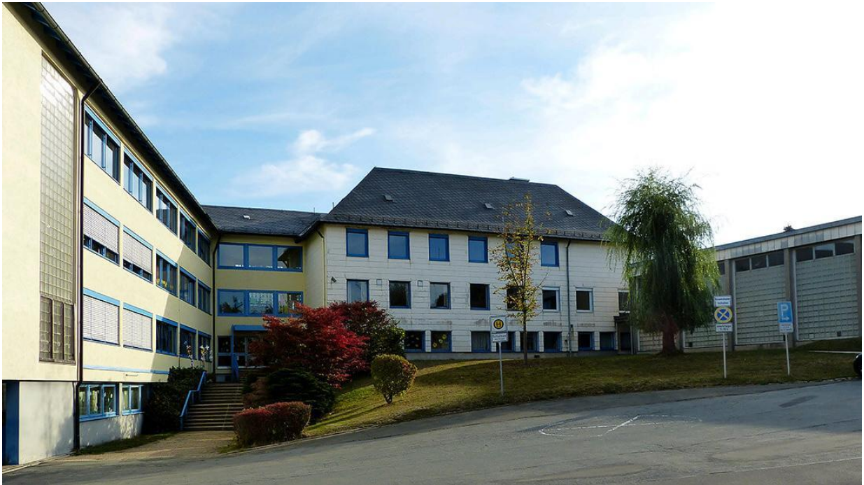
Figure 2: Schauenstein Elementary School (The Schauenstein City, 2023)
