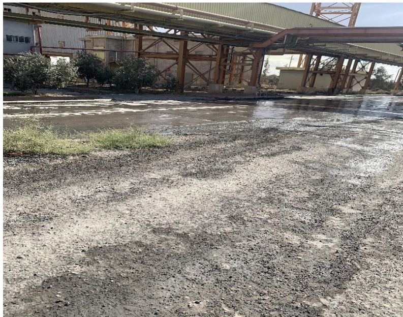
Figure 26, air-and-water spraying for dust control, (cementra jordan, n.d.)
