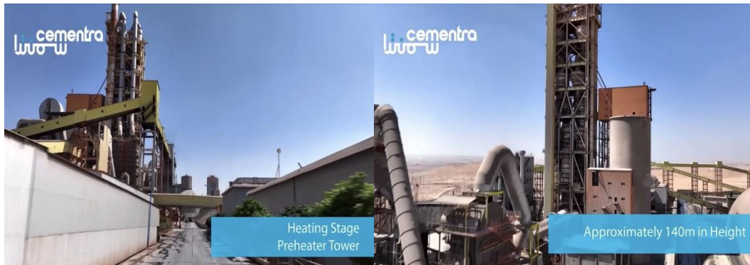
Figure 19, preheater tower, (cementra jordan, n.d.)
