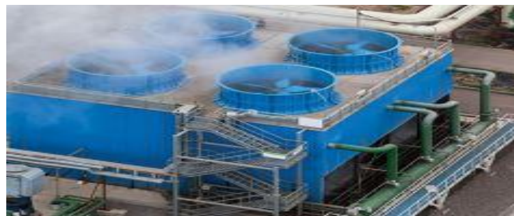
Figure 25, open recirculating cooling tower system, (Water, 2024)
