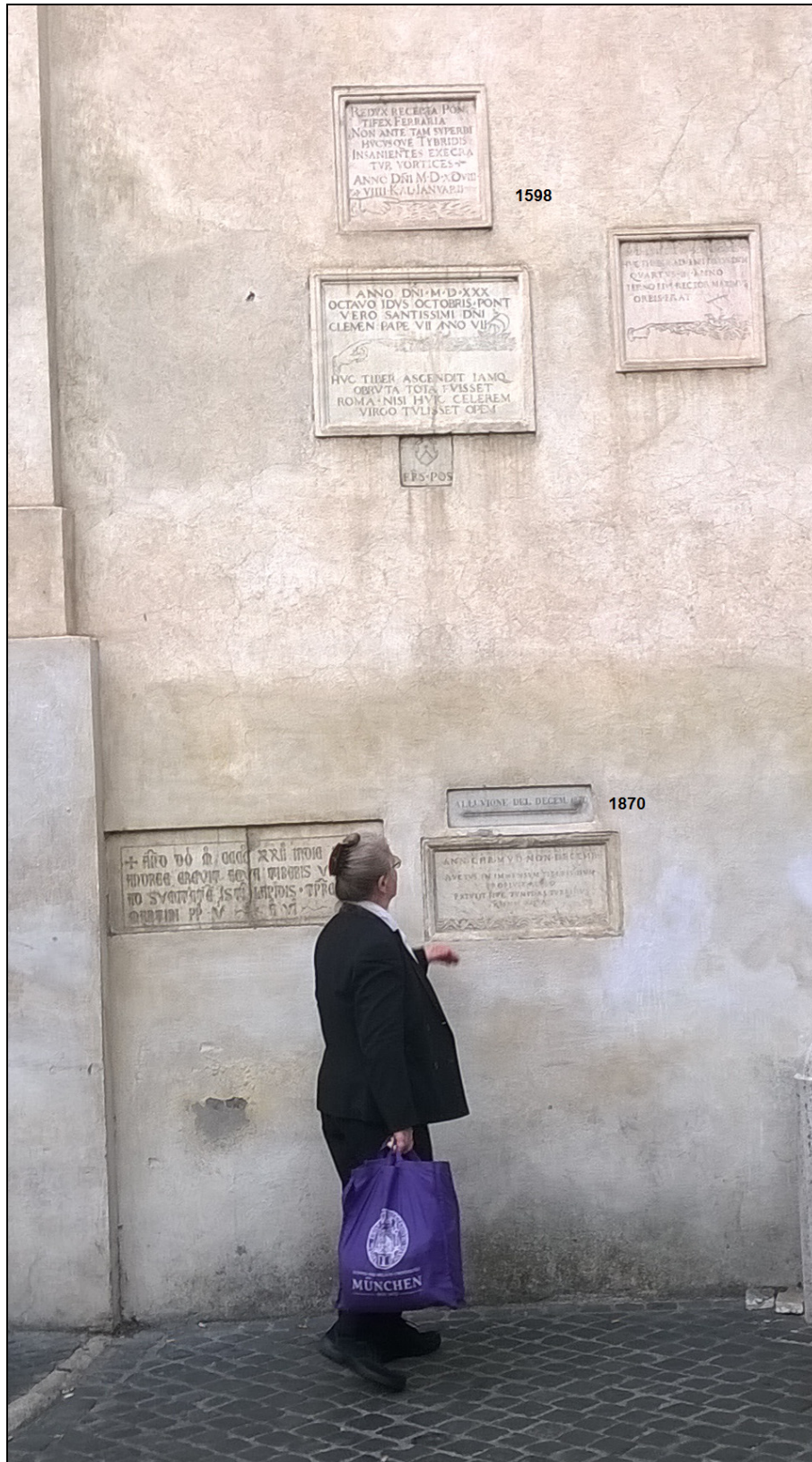
Fig. 10.2. Watermarks on the façade of the Church of S. Maria sopra Minerva in Rome, indicating the high waters of six post-antique Tiber floods (until 1870); cf. n. 149. Photo: Franz Xaver Schütz (September 2015). For the location of those watermarks, cf. Fig. 3.7 , labels: S. Maria sopra Minerva; Location of watermarks.
