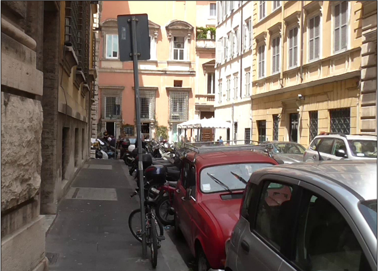
Fig. 3.2. The north-west corner of the junction of the roads Via in Lucina and Via del Giardino Theodoli, looking from south towards the incised corner of the former Palazzo Fiano-Almagià. Photo: F.X. Schütz (29-V-2016).
