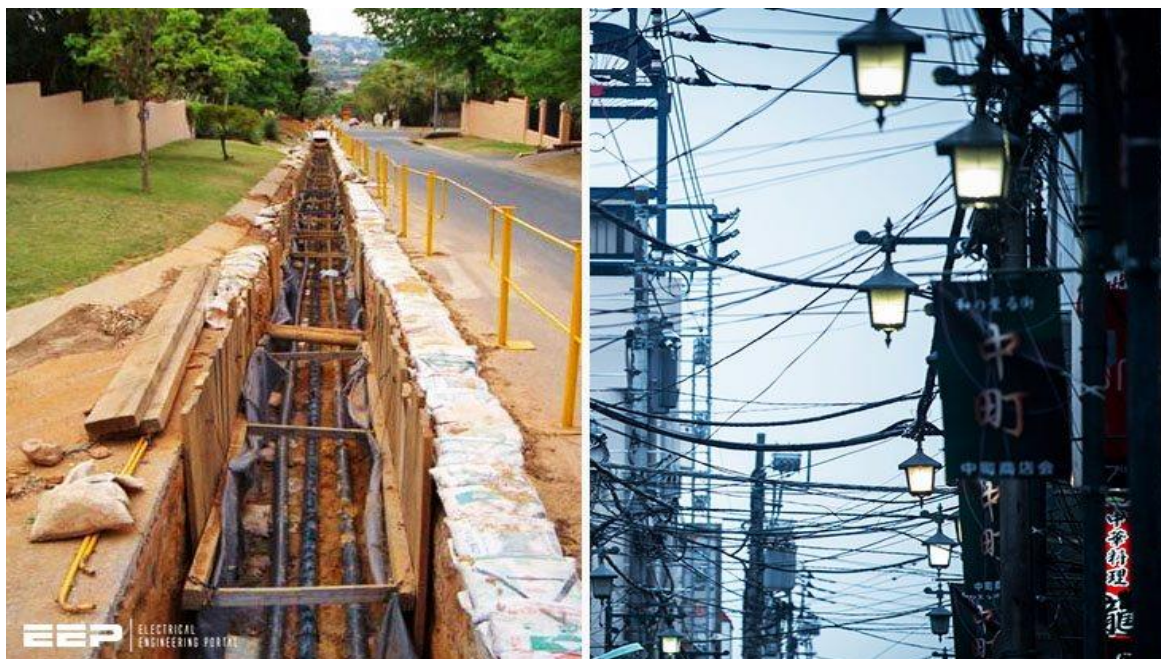
Figure 2. 4: Underground cables and overhead lines
