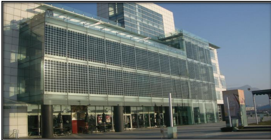
Figure 13: Building Integrated Photovoltaics [28]
