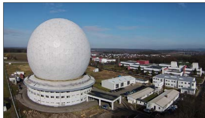
Fig. 1: Radom of the TIRA system at Fraunhofer FHR in Wachtberg, near Bonn
