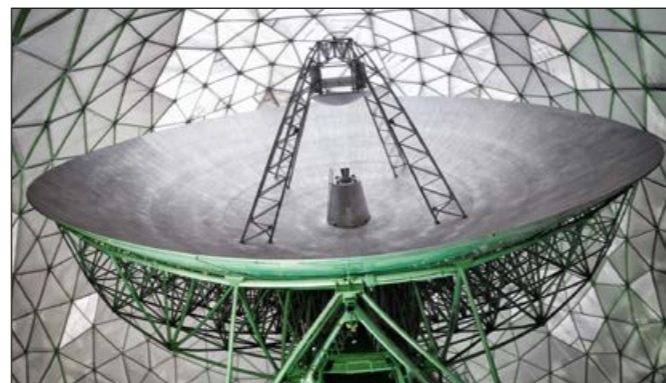
Fig. 2: The 34 m antenna of the TIRA system
