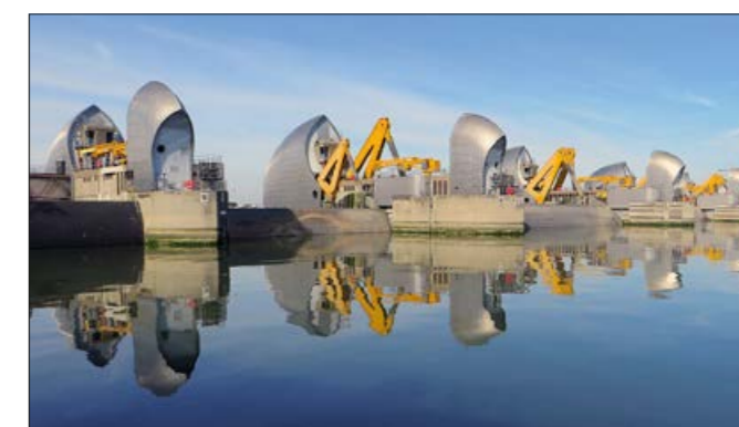
Fig. 4: Thames Barrier prevents the floodplain of most of Greater London from being flooded (Source: diamond greezer, https://www.flickr.com/ , CC BY-NC-ND 2.0, 08. 04. 2019)
