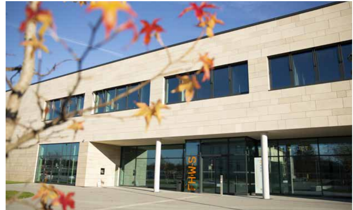
Neubau am Campus Ledward in Schweinfurt (Foto: S. Friese)
