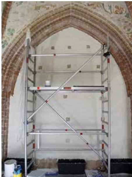
Figure 2: Application of desalination poultices
