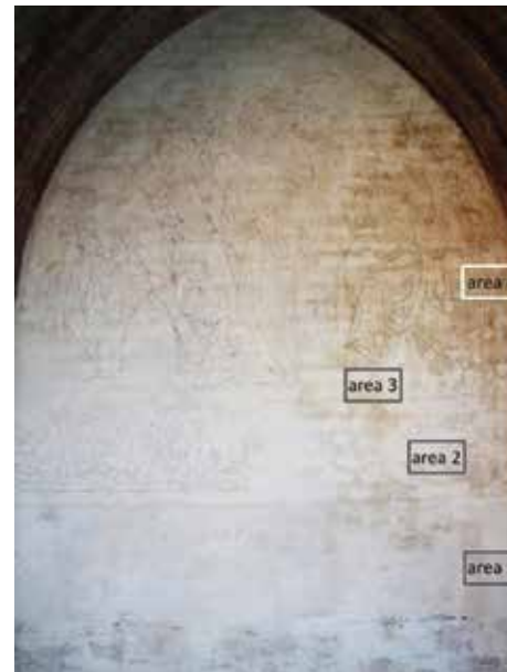
Figure 2: Bay no. 5, cloister of St. Peter Cathedral in Schleswig. Measurement areas 1 to 4 are depicted.
