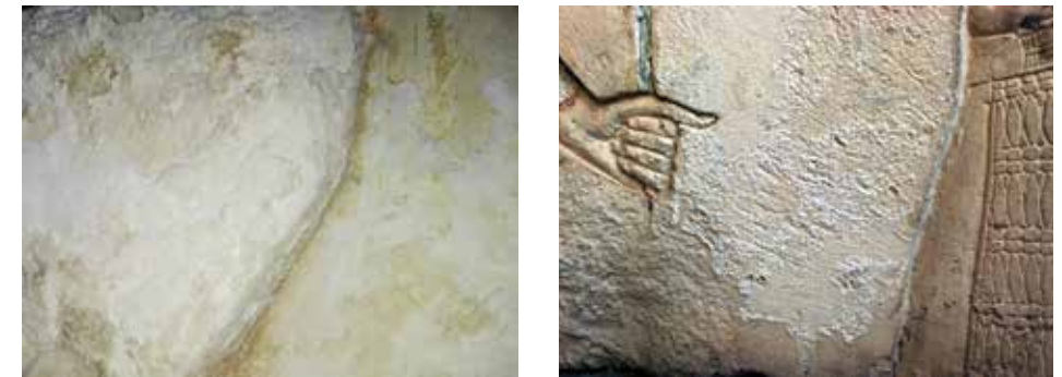
Figure 3: [left image] Crystallized salts in the upper area of the Ramesses II's side, [right image] Crystallized salts in the lower area of the same side.
