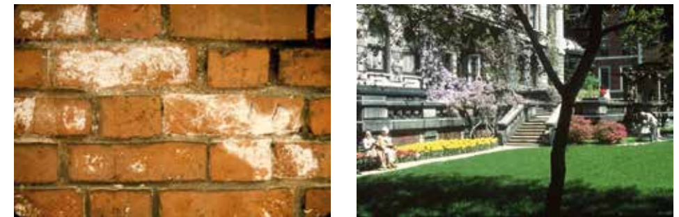
Figure 2: Detail of the brick wall showing the gypsum efflorescence formed on the parallel wall below grade to that seen in the garden at right.
