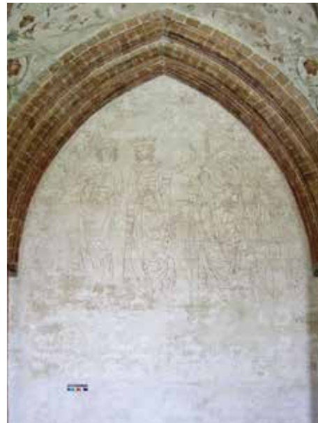
Figure 3: After the application of desalination poultices
