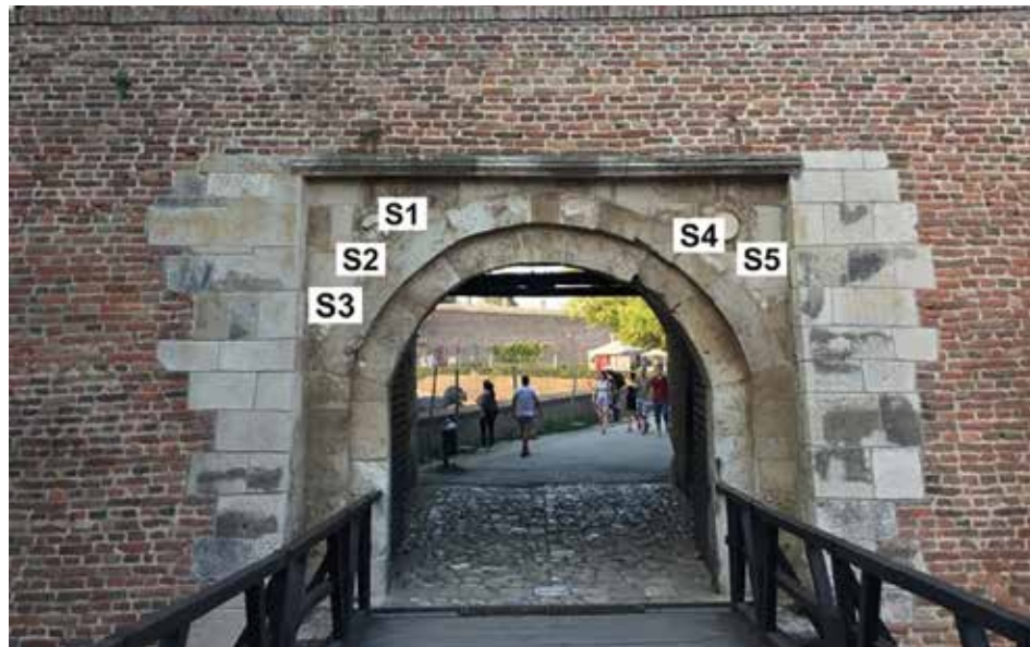
Figure 1: The view of the Karadjordje's Gate in Belgrade (Serbia) and position of the taken salt samples
