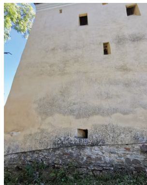
Fig. 30 (left) and Fig. 31 (right): The Northern wall – new cracks and humidity problems.
