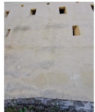
Fig. 30 (left) and Fig. 31 (right): The Northern wall – new cracks and humidity problems.
