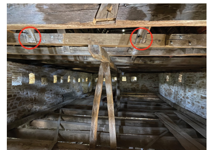
Fig. 5: Dovetail joint and overleafing.
