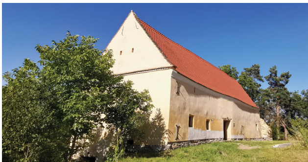
Fig. 21: The „Fruit-House“ from South-West – the curvature of the Southern wall is visible in the middle, above the entrance.
