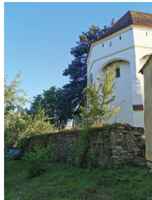
Fig. 26 (left) and Fig. 27 (right): The remains of the ring wall on the East side of the „Fruit-House“ – here the wall still plays a role in holding together the ground around the church.
