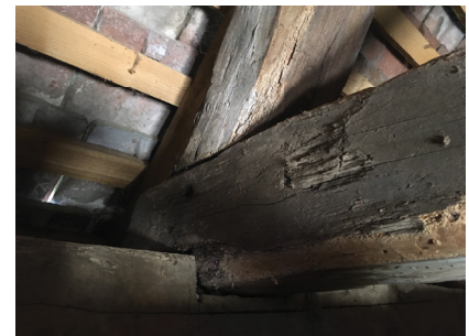
Fig. 6: Tongue between rafter and distorted beam.
