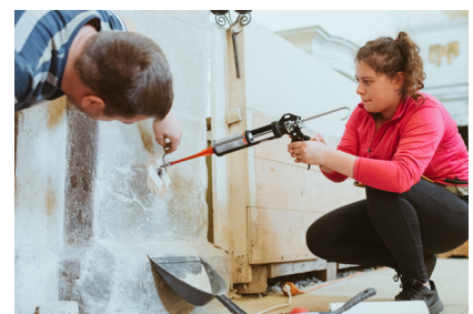
Fig. 4: Drilling the holes for the height bolts.
