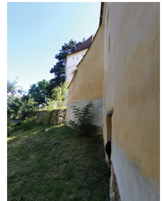
Fig. 26 (left) and Fig. 27 (right): The remains of the ring wall on the East side of the „Fruit-House“ – here the wall still plays a role in holding together the ground around the church.
