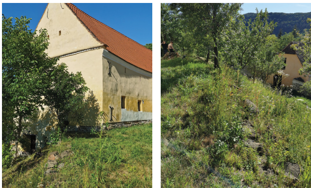
Fig. 22 (left) and Fig. 23 (right): The Fruit House from south-west and the remains of the first ring wall that used to flank the building from East and West.
