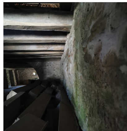
Fig. 13 (left): The Southern wall deformation
