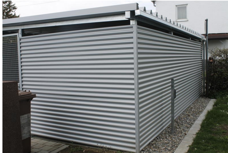
Figure 2.6. Corrugated iron sheets as facade elements [65]
