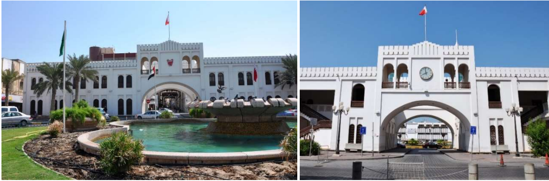
Fig. 3.3-16 and 3.3-17: Bab al-Bahrain and Customs Square after the refurbishment in the 1980s photographed in 2011. Source: Bahrain Authority of Culture and Antiquities
