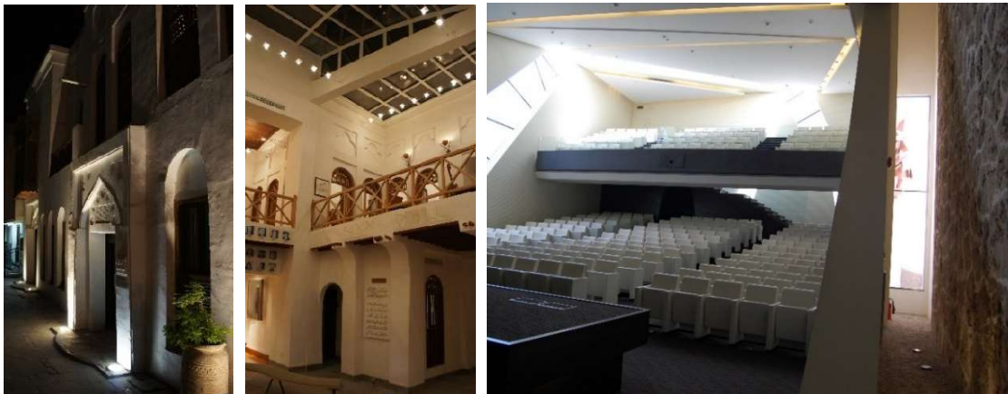
Fig. 3.2-13, 3.2-14 and 3.2-15: Exterior and interior views of Abdullah Al Zayed House and the auditorium of Shaikh Ebrahim Centre in Muharraq in 2014. Photos: Nils Schinker and Eva Battis (right)
