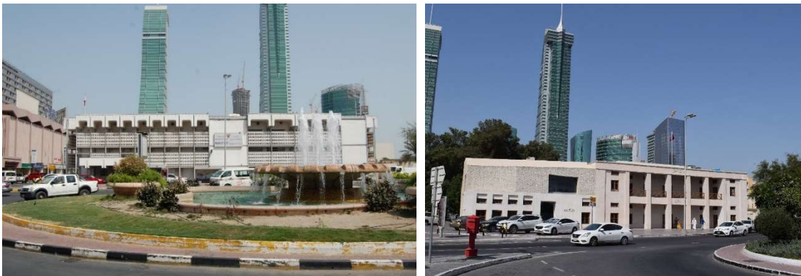
Fig. 3.3-28 and 3.3-29: The Customs House in 2014 and after its restoration and extension in 2023. Photos: Eva Battis
