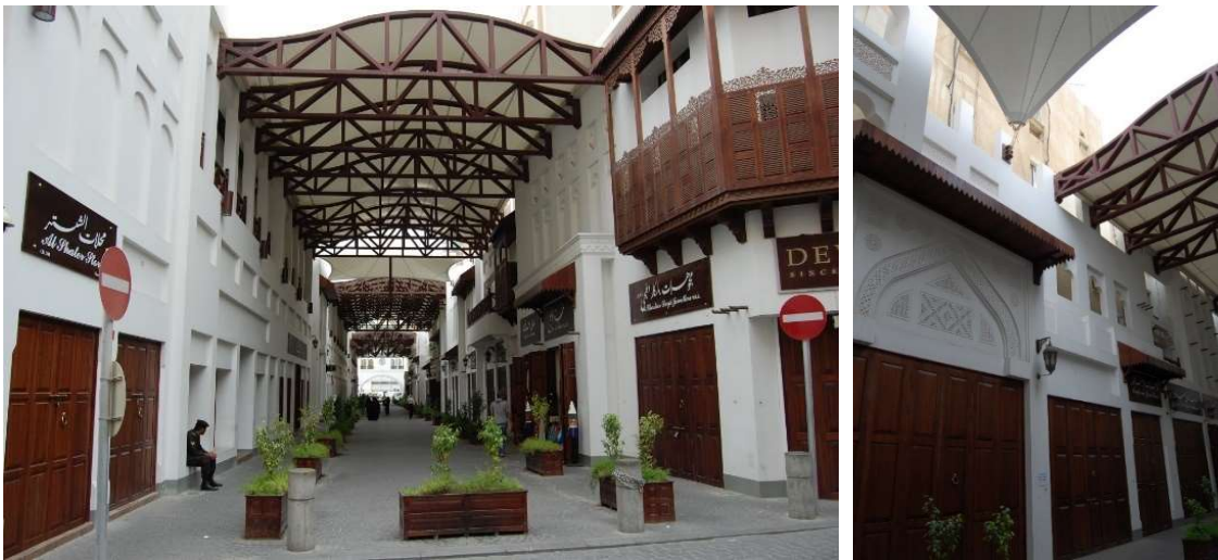
Fig. 3.3-19 and 3.3-20: Bab al Bahrain Avenue and detail of the screen façade in 2011. Photos: Eva Battis
