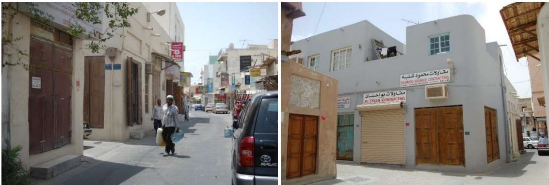
Fig. 3.4-17 and 3.4-18: The western Siyadi Shops on Tujjar Avenue after the façade works in 2012. Photos: Eva Battis
