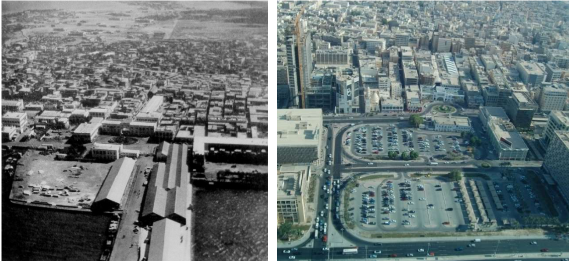
Fig. 3.3-2 and 3.3-3: Aerial view of the site from the north in the early 1950s and in 2012. Source (left): Belgrave 1975 [1953], 109; Photo (right): Eva Battis
