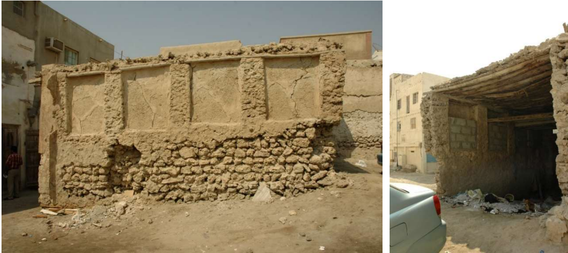
Fig. 3.4-11 and 3.4-12: The sixth shop unit before rehabilitation in 2008. Photos: Eva Battis
