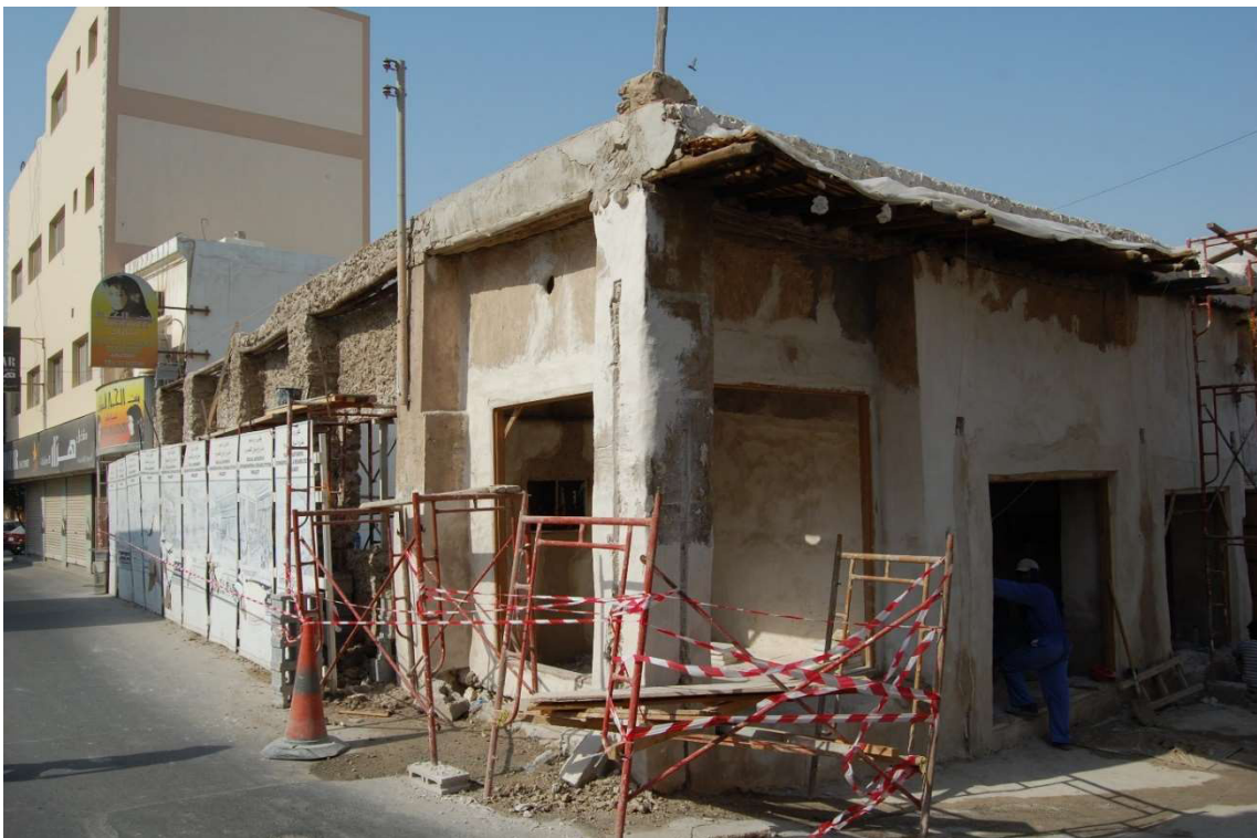
3.4.1 – 41: Eastern elevation along Bu Maher Avenue during reconstruction and restoration in 2011.
