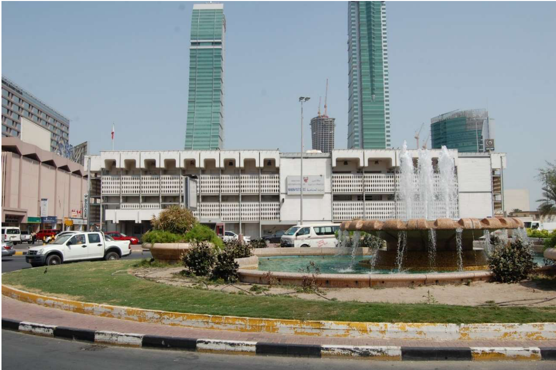
3.3.1 – 12: Southern elevation with added façade element and Bab al-Bahrain roundabout in 2014.
