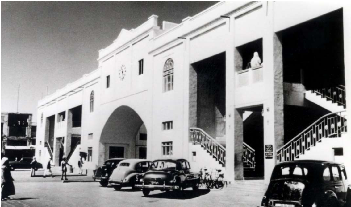
3.3.1 – 23: Southern elevation of Bab al-Bahrain viewed from the south-east in the 1950s. Source: Bahrain Authority for Culture and Antiquities
