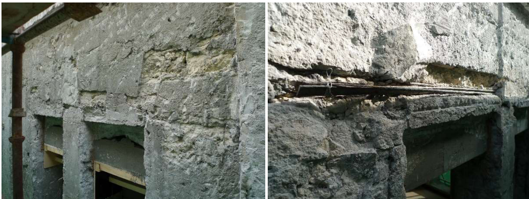
3.3.1 – 51 and 52: Details on exterior wall and window lintels after invasive investigations (heightened and arched in the 1980s) during works in 2011 (straightening and lowering the lintels)
