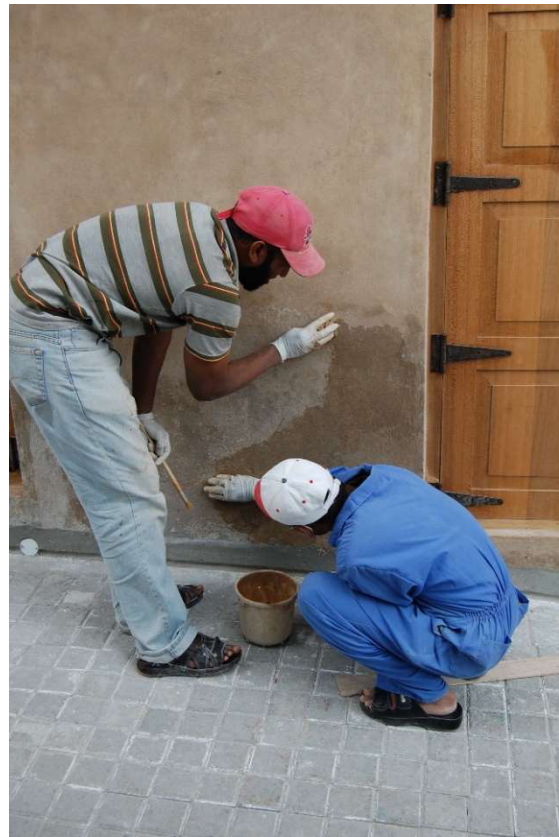
3.4.1 – 58 and 59: Reconstruction of a coral stone wall in 2011 (left) and pigmentation works on new traditional surface plaster of a northern shop unit in 2012
