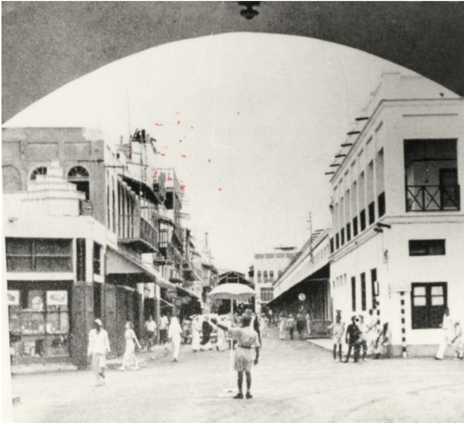
3.3.1 – 74: View along Barrett Avenue from Bab al-Bahrain in the 1950s. Source: Bahrain Authority for Culture and Antiquities
