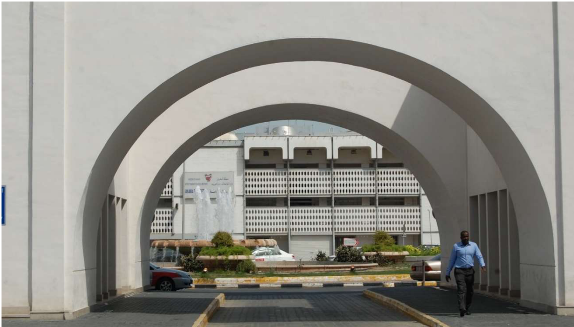
3.3.1 – 49: View of the Customs House through the arches of Bab al-Bahrain in 2014. Photos: Eva Battis
