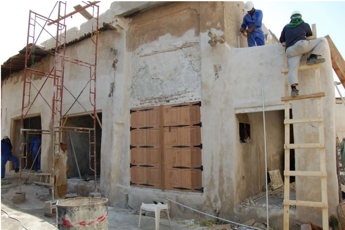
3.4.1 – 42: Northern elevation during restoration in 2011.
