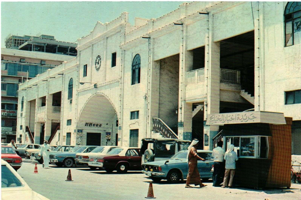
3.3.1 – 26: Southern elevation of Bab al-Bahrain in the 1970s. Source: Historic postcard, Battis personal archive
