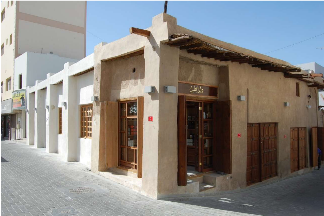
3.4.1 – 67: Northern and eastern elevation of the eastern Siyadi Shops in 2012.
