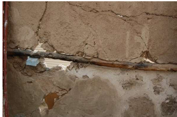
3.4.1 – 65 and 66: Coral stone masonry after deep filling and repointing (left) and coral stone slab ( farush ) wall masonry of the one-storeyed western Siyadi Shops during restoration in 2012.
