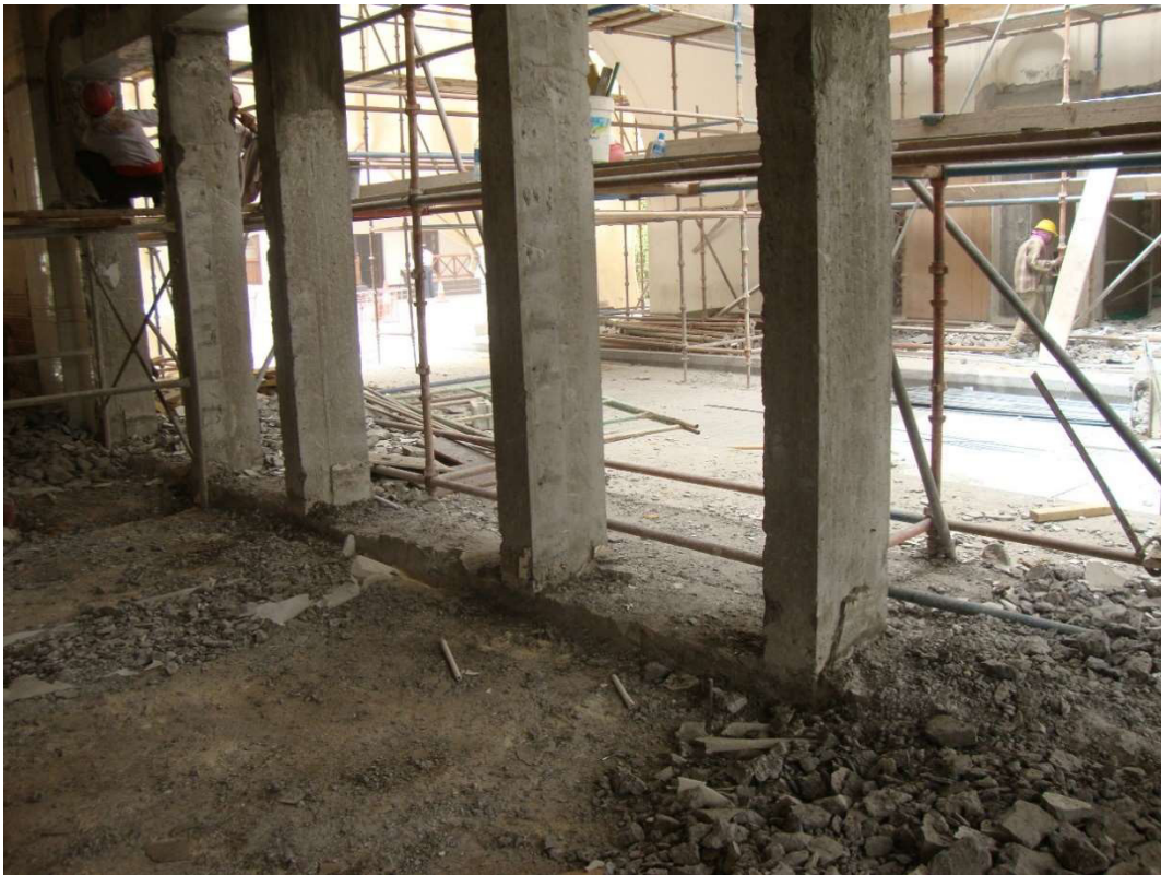
3.3.1 – 50: Uncovering the columns in the walls flanking the central gateway in 2011.
