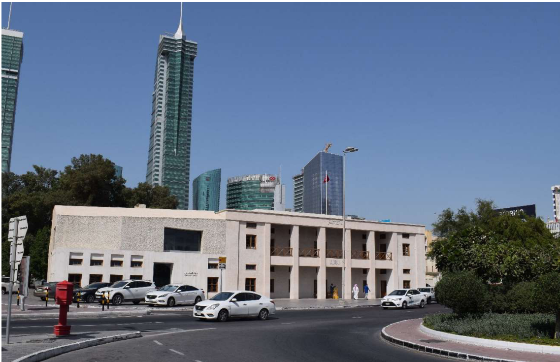
3.3.1 – 20: Southern elevation following the building's restoration and extension, 2023. Photo: Eva Battis
