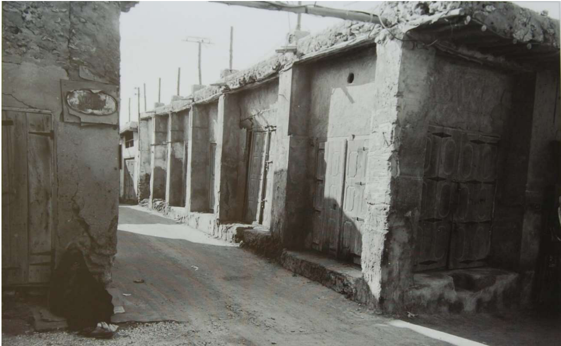
3.4.1 – 8: Historic view along Bu Maher Avenue with the Siyadi Shops Source: Al-Khan 2007, 90
