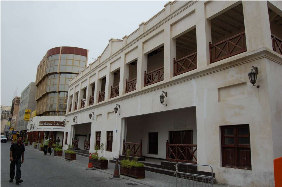
3.3.1 – 65: Northern elevation of the Post Office and Police Station viewed from the North-West after restoration in 2011.
