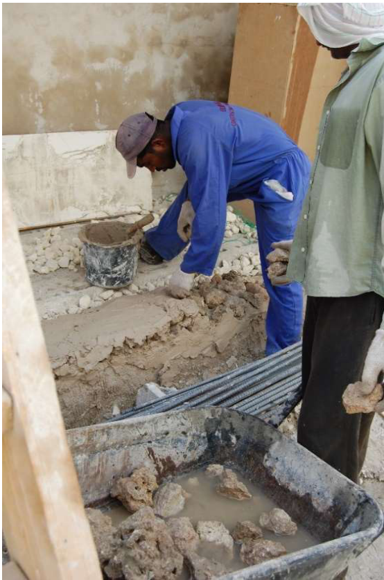
3.4.1 – 58 and 59: Reconstruction of a coral stone wall in 2011 (left) and pigmentation works on new traditional surface plaster of a northern shop unit in 2012
