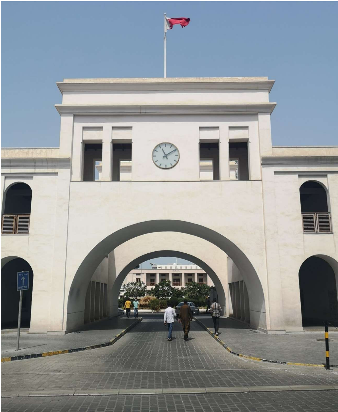
3.3.1 – 57: View of the restored Customs House through the arches of Bab al-Bahrain in 2021. Photo: Melanie Münzner
