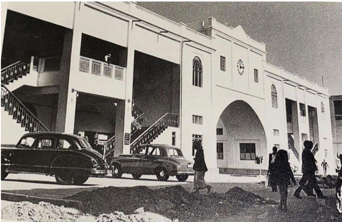
3.3.1 – 24: Southern elevation of Bab al-Bahrain viewed from the south-west in the 1950s. Source: Bahrain Authority for Culture and Antiquities
