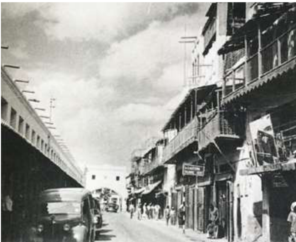
3.3.1 – 75: View along Barrett Avenue towards Bab al-Bahrain with Government Shops and Offices before the addition of the upper floor. Source: Bahrain Authority for Culture and Antiquities
