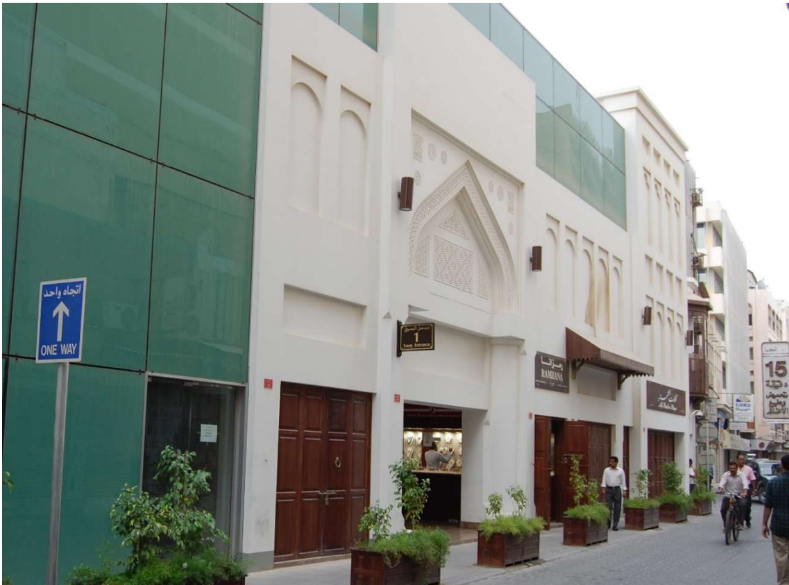
3.3.1 – 87: Southern elevation of the mall building in 2011.
