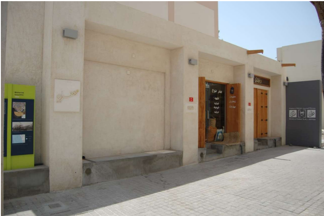
3.4.1 – 77: Westwards view along the pedestrian lane with newly constructed shop units in 2012.
