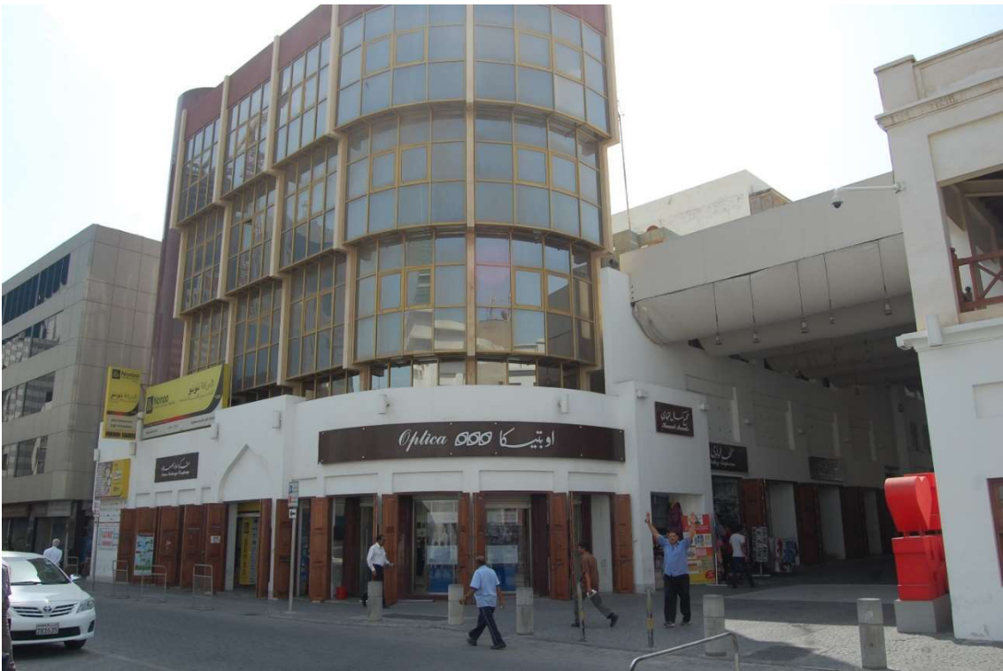
3.3.1 – 98: Detail view of the screen façade along Bab al-Bahrain Avenue at the junction with Al Khalifa Avenue in 2014, Photos: Eva Battis
