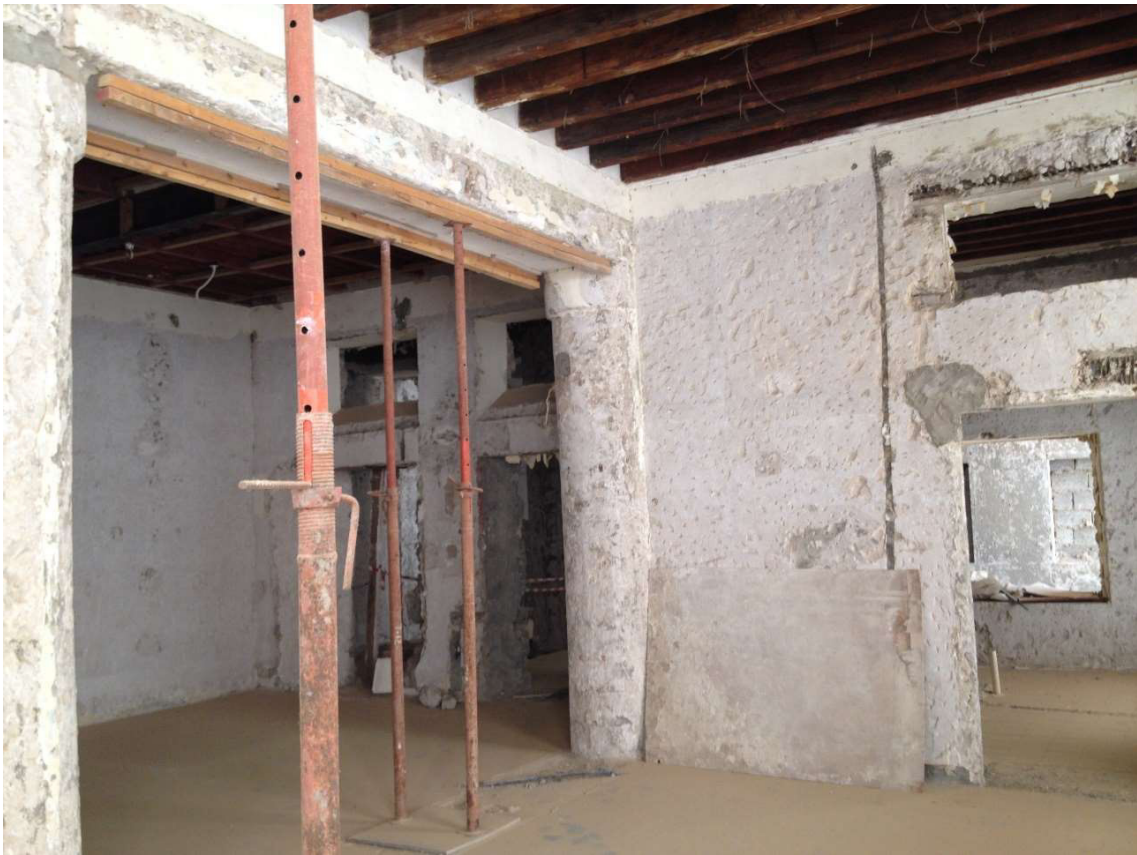
3.3.1 – 17: View of the first-floor interior during restoration in 2015.
