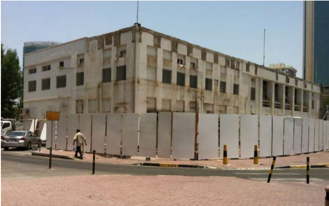
3.3.1 – 15: Western and southern elevations during restoration in 2015.
