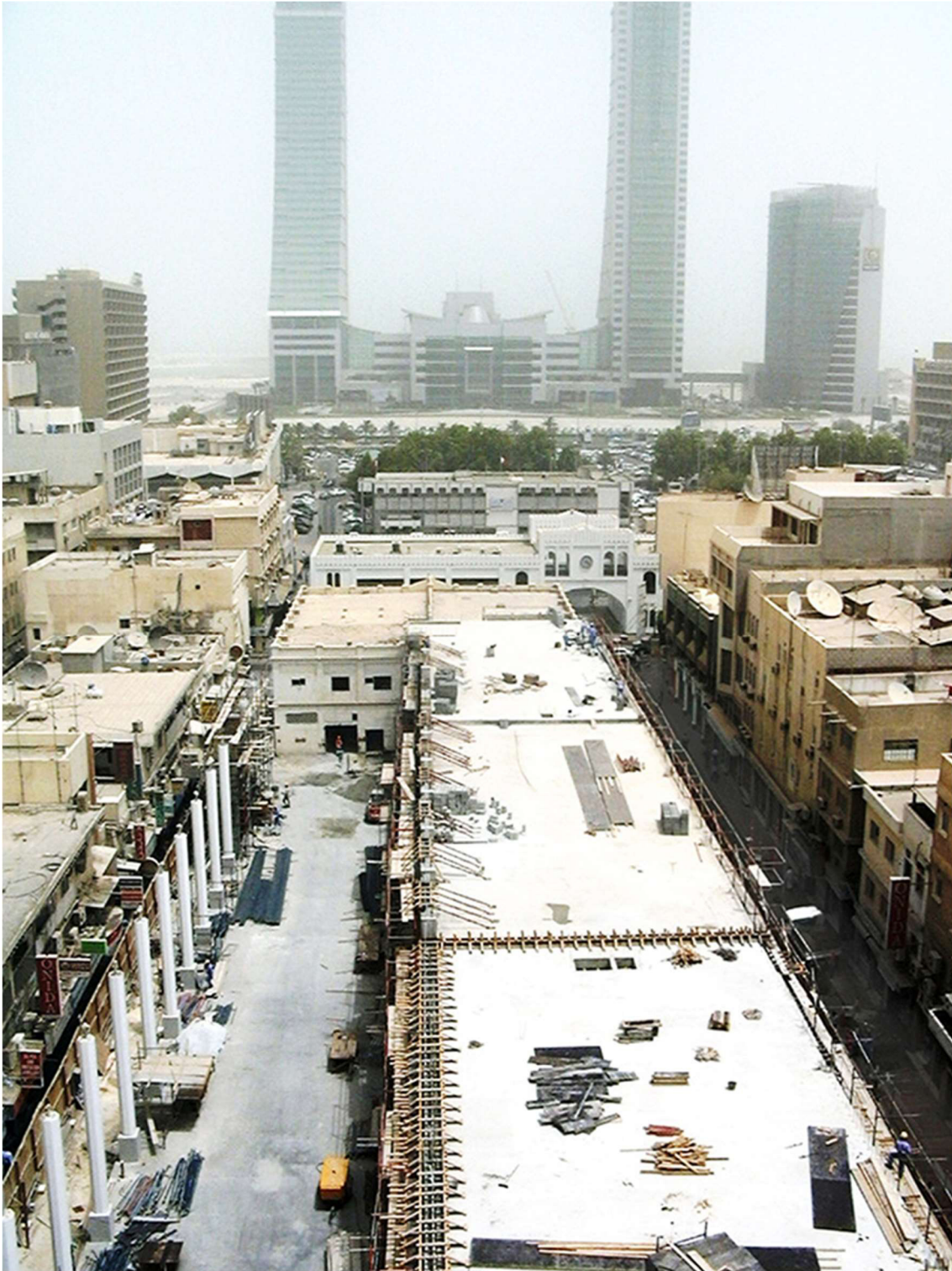
3.3.1 – 79: Aerial view of the mall building during construction in 2009.
