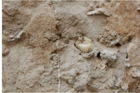
3.4.1 – 63 and 64: Details of coral stone masonry with palm trunk (left) and during deep filling of the coral stone masonry of the one-storeyed western Siyadi Shops in 2012.
