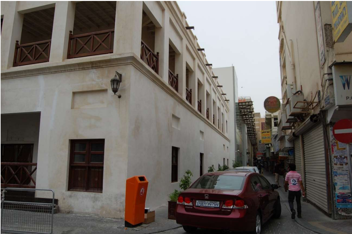
3.3.1 – 66: View northwards along Al-Mutanabi Avenue with western elevation of Post Office and Police Station in 2011. Photos: Eva Battis
