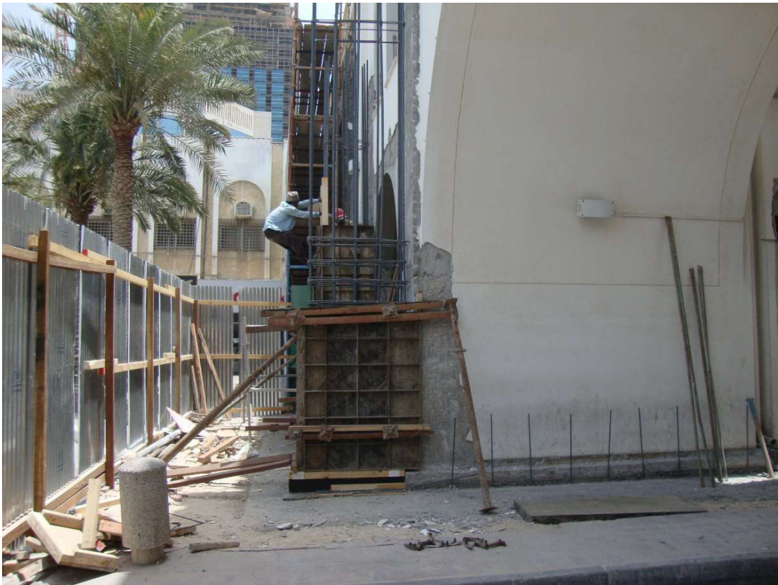
3.3.1 – 56: Construction of the protruding risalite in 2012. Source photos: Plan Architecture & Design
