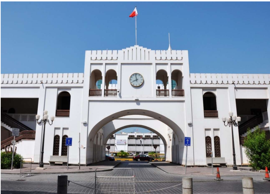
3.3.1 – 35: Southern elevation of Bab al-Bahrain after refurbishment of the 1980ies photographed in 2011. Source: Bahrain Authority for Culture and Antiquities
