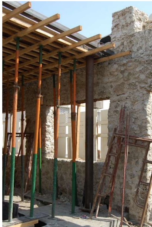
3.4.1 – 51 and 52: Reconstructed eastern wall along Bu Maher Avenue and roof of the café space under construction in 2011.
