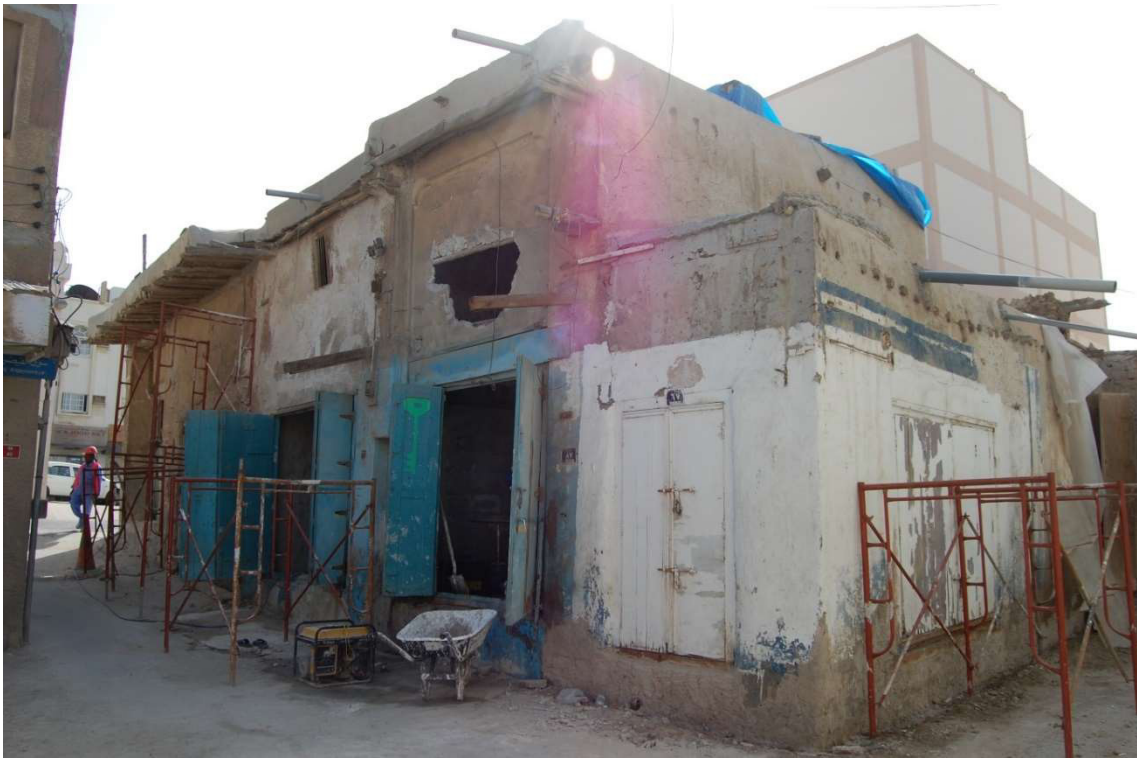
3.4.1 – 40: Northern and western elevations during restoration in 2011.
