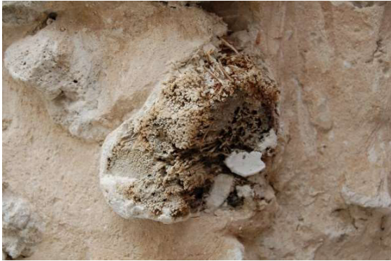
3.4.1 – 63 and 64: Details of coral stone masonry with palm trunk (left) and during deep filling of the coral stone masonry of the one-storeyed western Siyadi Shops in 2012.
