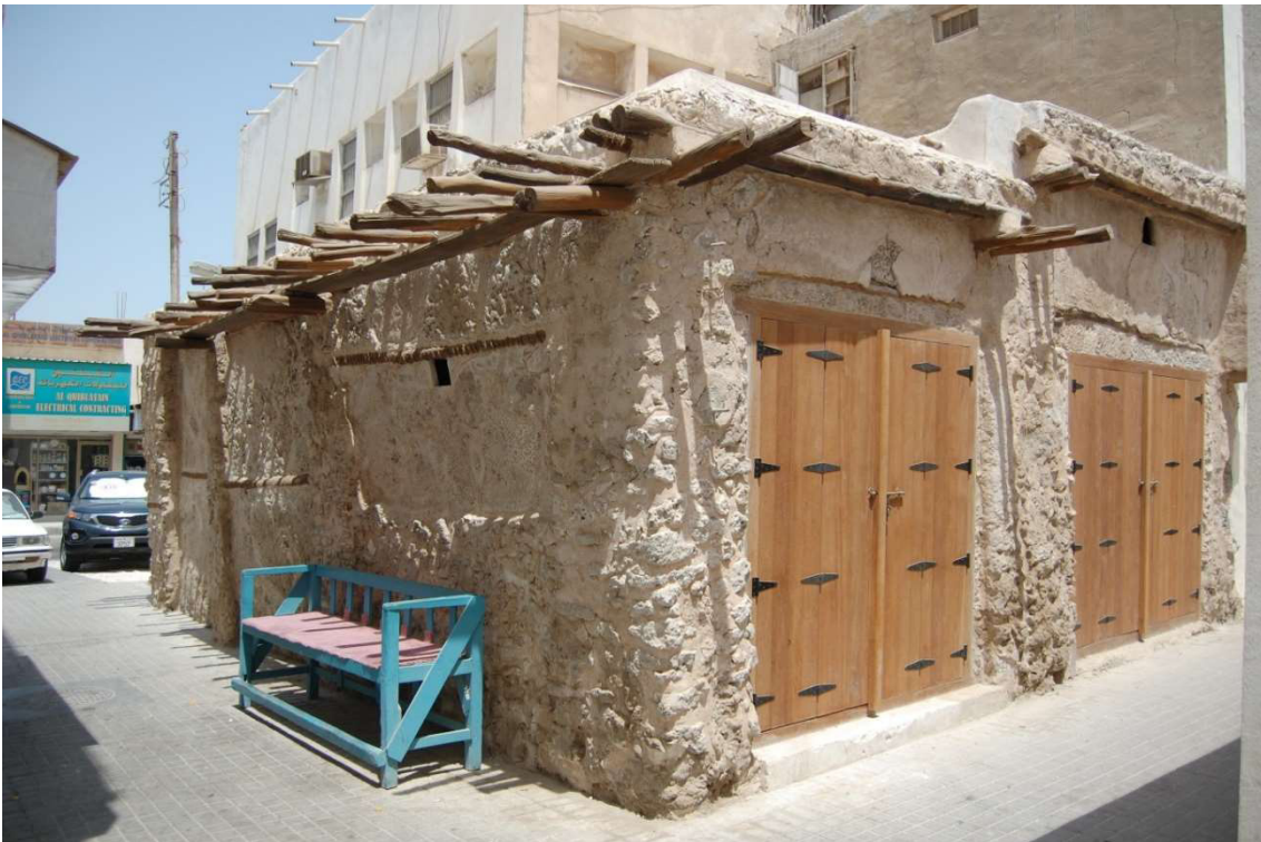
3.4.1 – 82: The one-storeyed units of the western block viewed from the pedestrian lane in 2012.
