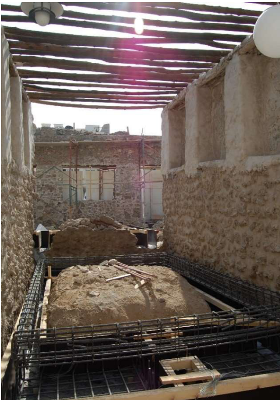
3.4.1 – 46 and 47: Lower café space during (2011) and after (2012) the installation of reinforced concrete foundations and floor tiles.
