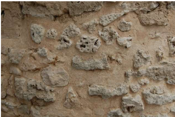
3.4.1 – 65 and 66: Coral stone masonry after deep filling and repointing (left) and coral stone slab ( farush ) wall masonry of the one-storeyed western Siyadi Shops during restoration in 2012.
