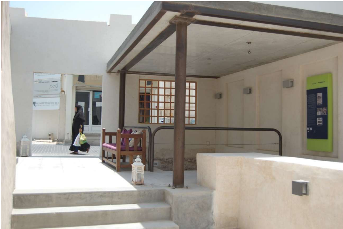
3.4.1 – 73: Westwards view of the outdoor space in 2012.
