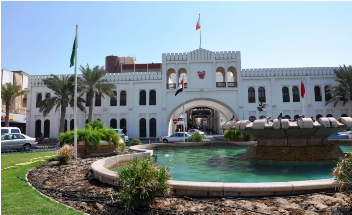
3.3.1 – 34: Northern elevation of Bab al-Bahrain after refurbishment of the 1980ies photographed in 2011. Source: Bahrain Authority for Culture and Antiquities
