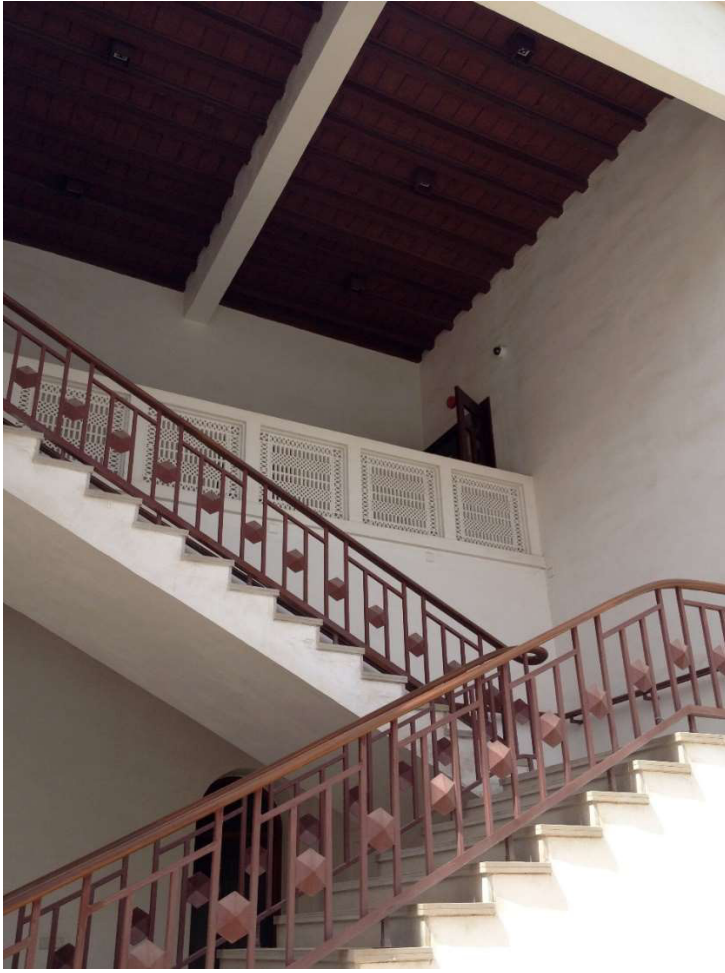
3.3.1 – 48: Detail view of the western staircase in the southern elevation of Bab al-Bahrain in 2015.
