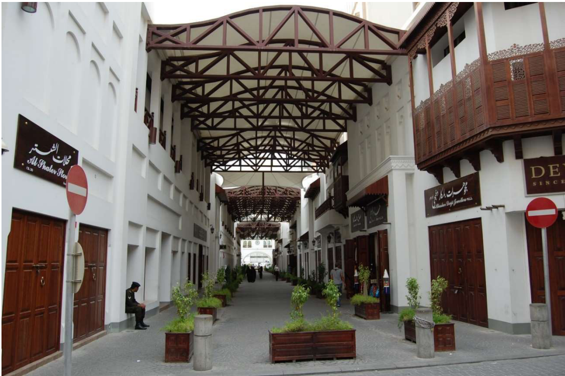
3.3.1 – 80: View to the north along Bab al Bahrain Avenue in 2011 with the screen façade element on the right and the mall building on the left.
