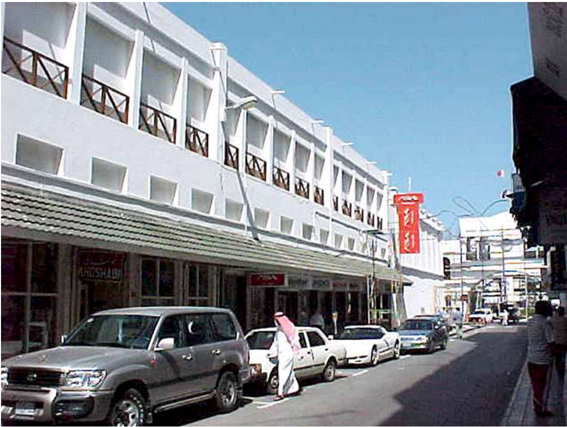
3.3.1 – 78: Government Shops and Offices viewed from the south in 2004. Source: https://www.archnet.org/sites/15785?media_content_id=114199 (accessed June 29, 2022)
