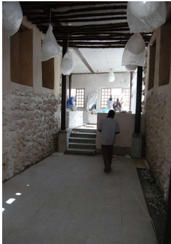
3.4.1 – 46 and 47: Lower café space during (2011) and after (2012) the installation of reinforced concrete foundations and floor tiles.
