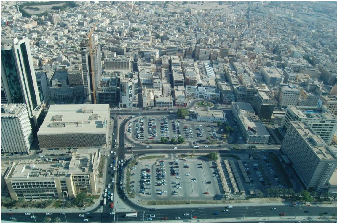
3.3.1 – 2: View southwards of Manama and Bab al-Bahrain area from Financial Harbor with King Faisal Highway in the forefront, October 2012.
