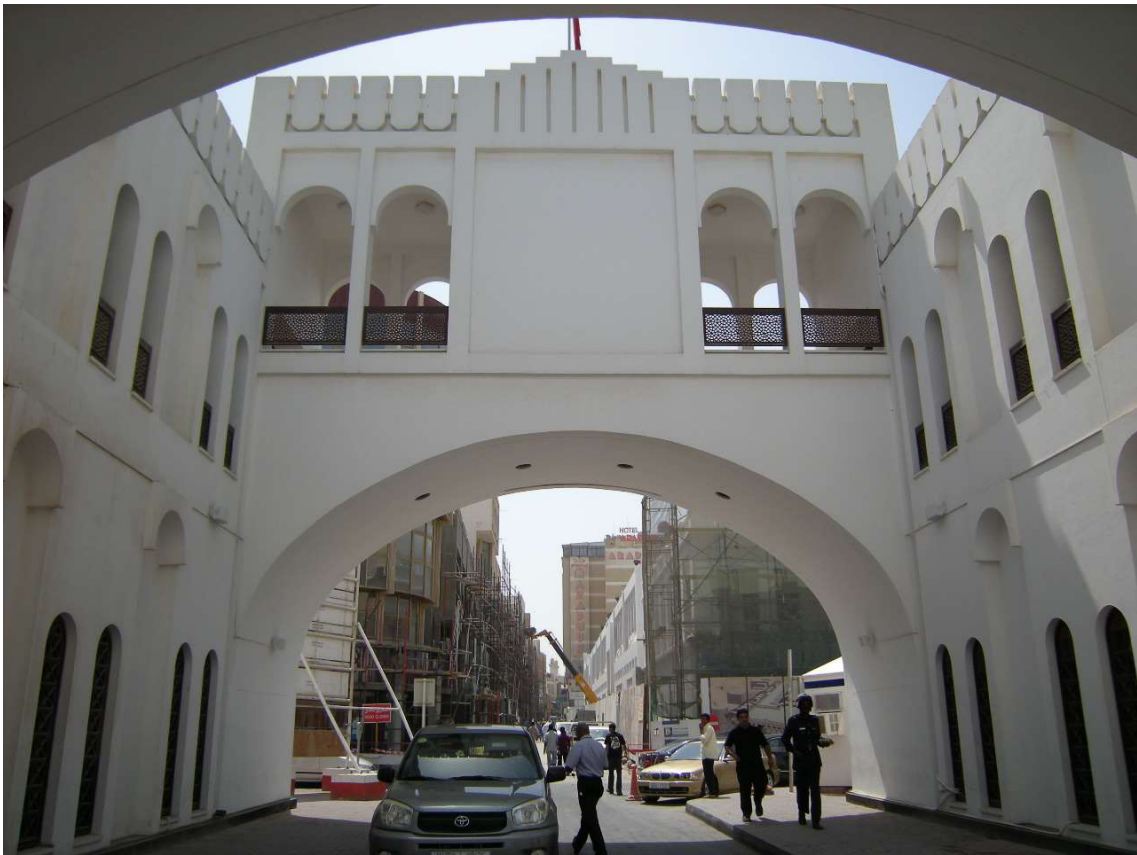
3.3.1 – 36: View from Bab al-Bahrain to the south during construction works at Bab al-Bahrain Avenue in 2009.
