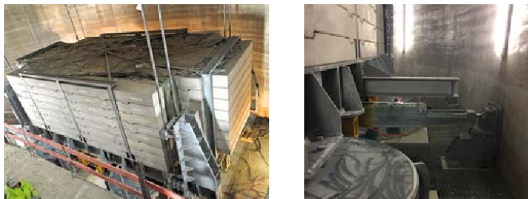
Figure 2.5: TMD in Rottweil Test Tower (Left: Pendulum rope supported TMD mass, Right: Linear Motor as actuator) 11 .
