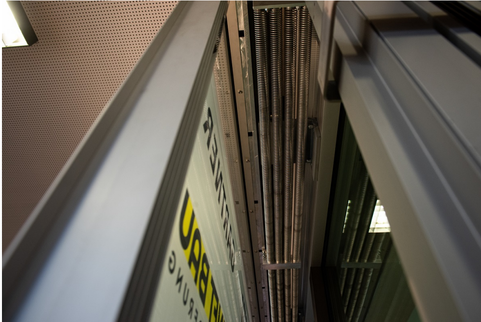
Figure 7.8: Spring system of the moveable DSF (Source: Ralf Schuster, BTU Cottbus-Senftenberg).
