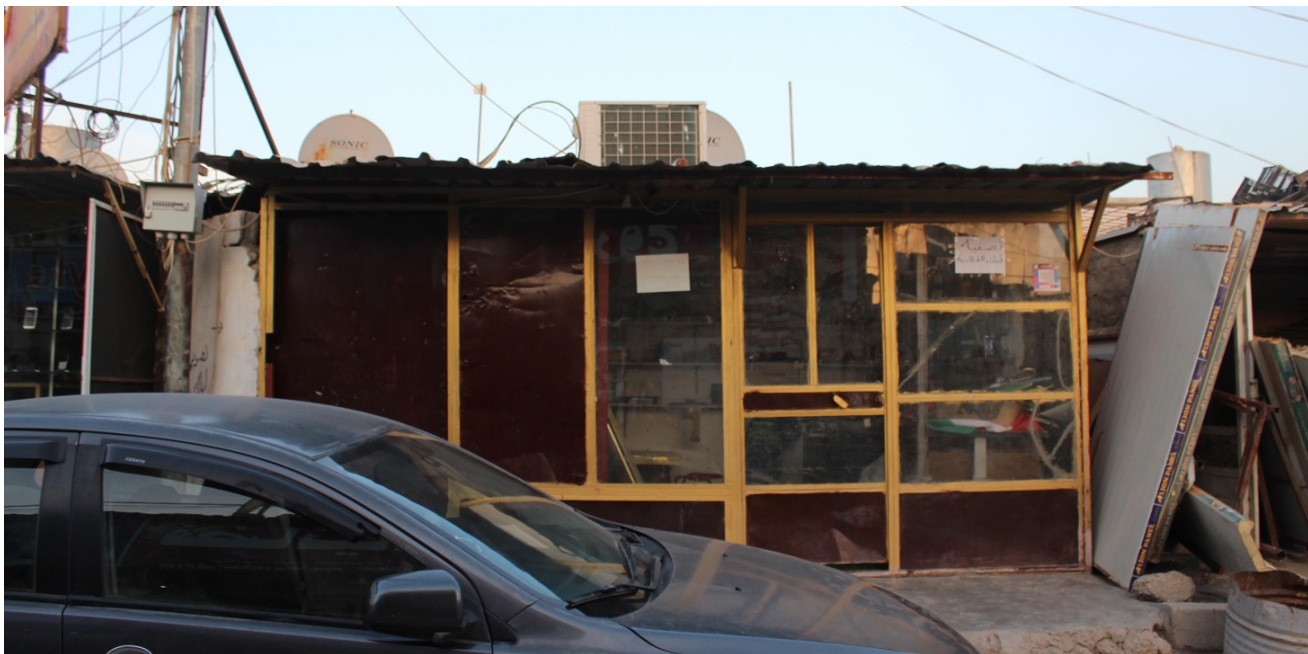
Abu Sipan’s Shop 2 façade. It is used as a school stationery, and rented to “an old friend” from Qamishli.. on the right side of the picture, you can see the sandwich panel roof that Abu Sipan will add to one of the rooms (Author, 2018)
