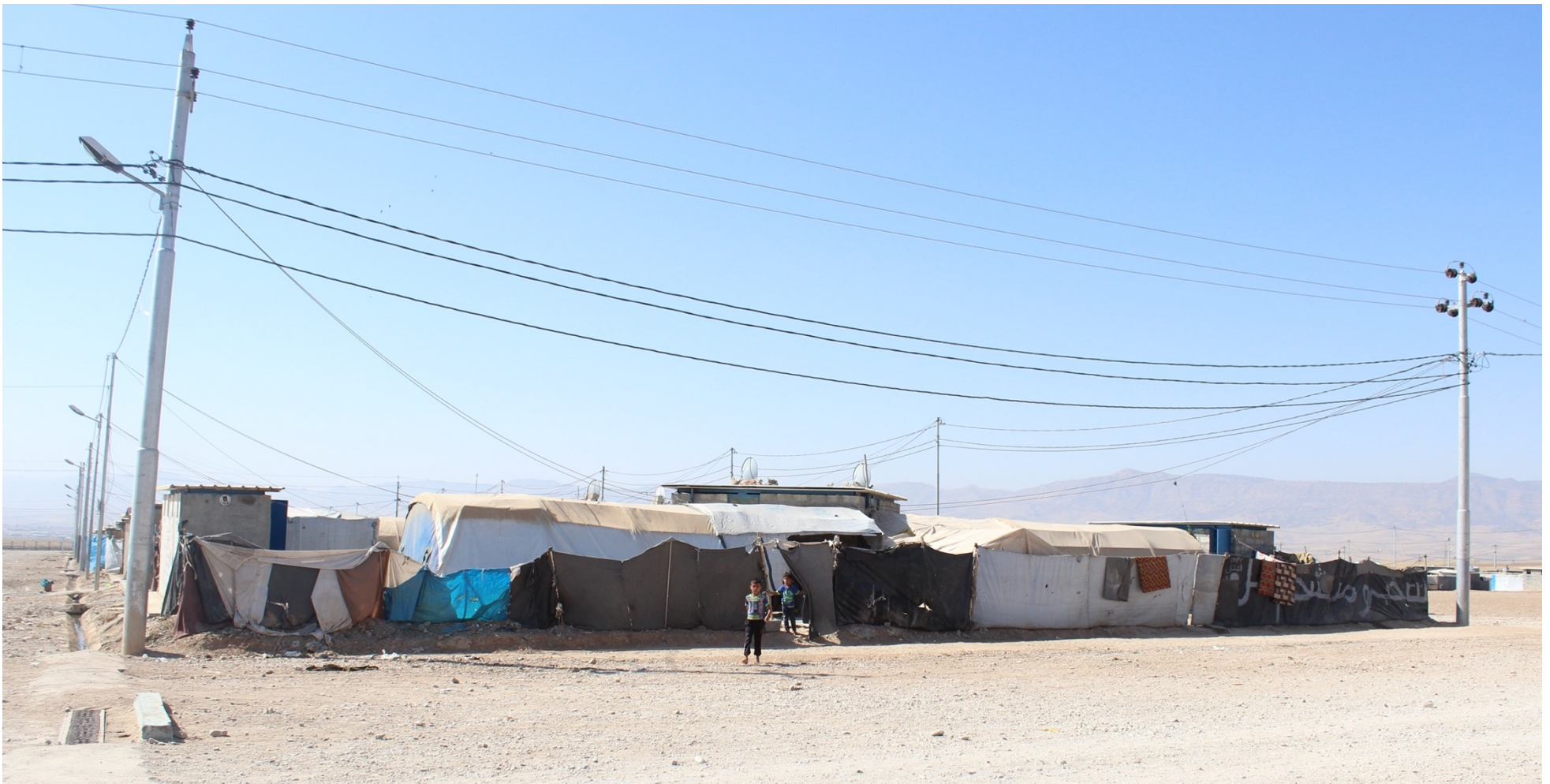
Ashti IDP Camp showing the improved shelter setting with the brick-built utilities, patched up fabrics of improvised spatial practices. The iron-grid layout demarcated by the lamp posts. The roads are cleared but
