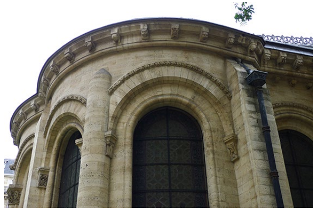
Fig. 12: Advanced stereotomy in the abbey church of Saint-Martin-des-Champs in Paris, first half of twelfth century
