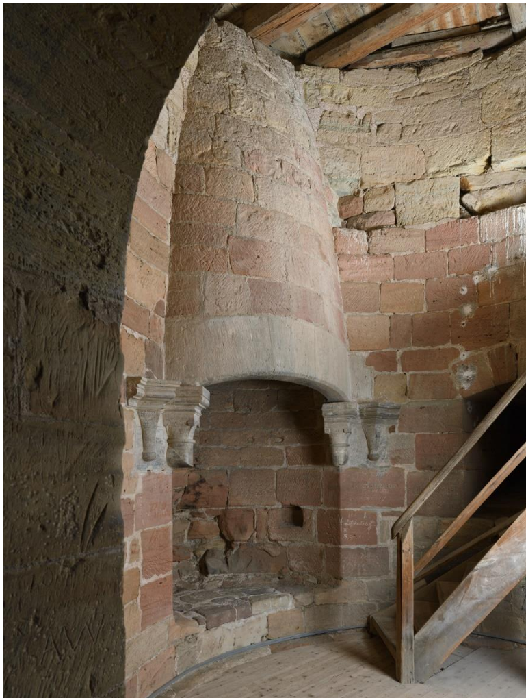
Fig. 1. Fireplace in the first storey viewed from the entering corridor. (R. Wieczorek)
