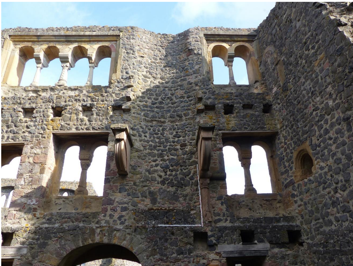
Fig. 5. North wall of the palace (Palas) at Münzenberg castle (1170). The remains of the chimney flue and Mantelpiece reaching trough two storeys dominate the wall. (author)
