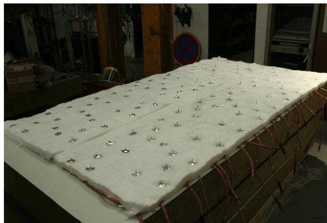
Figure 3.4. Applying insulation materials to avoid temperature loss [8]
