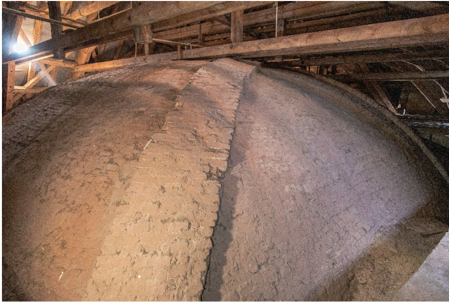
Fig. 06: The extrados of the main vault, north-east corner
