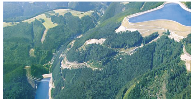
Figure 3 – View of the two reservoirs of the Plant in Goldisthal [13]
