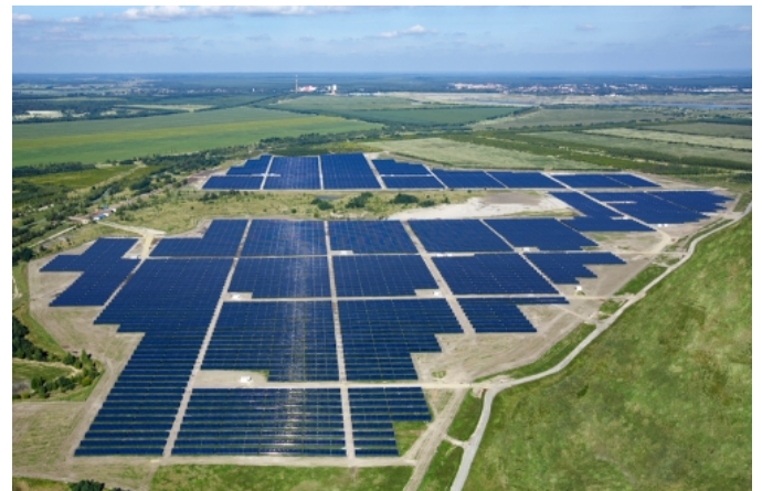
Figure 4: Senftenberg Solar Park, Phoenix Solar Group
