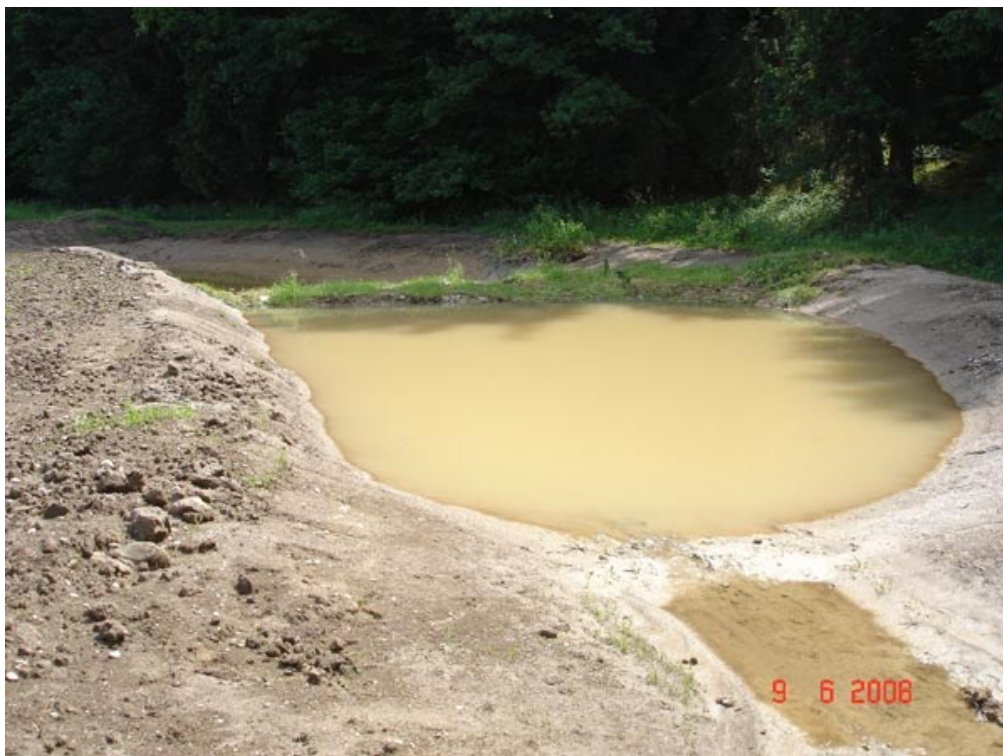
Fig. 25: Sediment trap at a brook in Bavaria/Germany (source: Bavarian Ministry of Nutrition, Agriculture and Forests)
