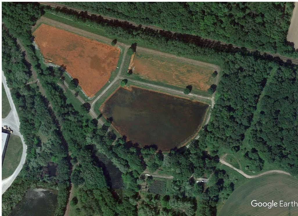
Fig. 23: Oxidation and sedimentation ponds of the water treatment system at Eichower Fließ
