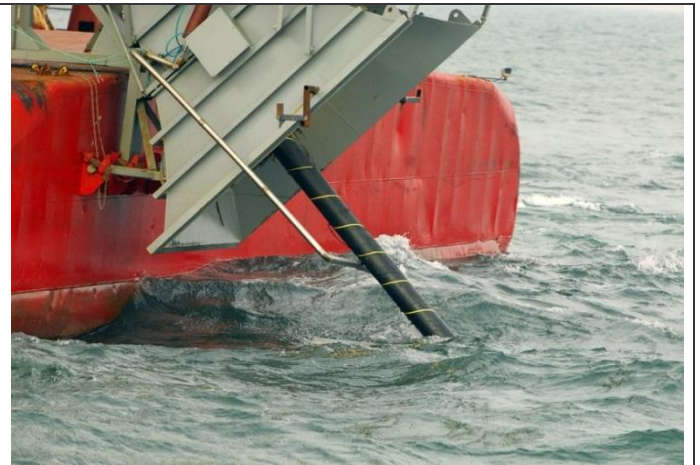
Fig. 14: Laying of HVDC lowered into the sea [15]
