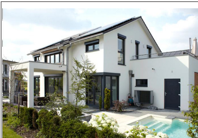
Plus energy house. Besides of solar plants and ventilation system you can't make out any optical differences to normal houses.
