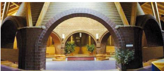
Figure 7. Kindergarten Sorsum, vault made of loam bricks [9]
