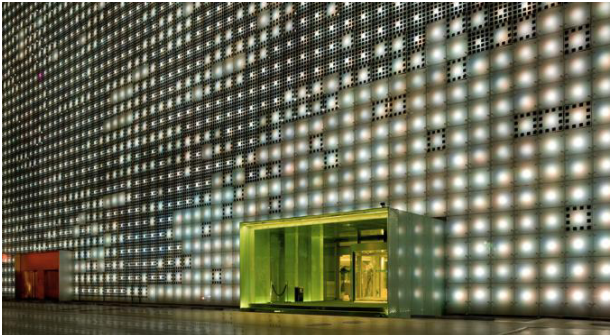
Figure 10: Greenpix, in Beijing, Simone Giostra & Partners Architects (20)
