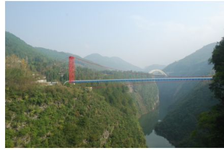
Figure 7: Picture of Yesanhe cross-cliff river pipeline-bridge
