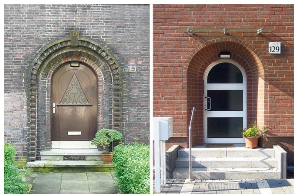
Figure 10. Energetic redevelopment of a housing estate in Dortmund, Germany. Entrance of Kronprinzenstraße 129 before and after. The left side shows unpretentious ornaments and patina on the facade. On the right side the former charm is covered under insulation packaging and brick imitation.
