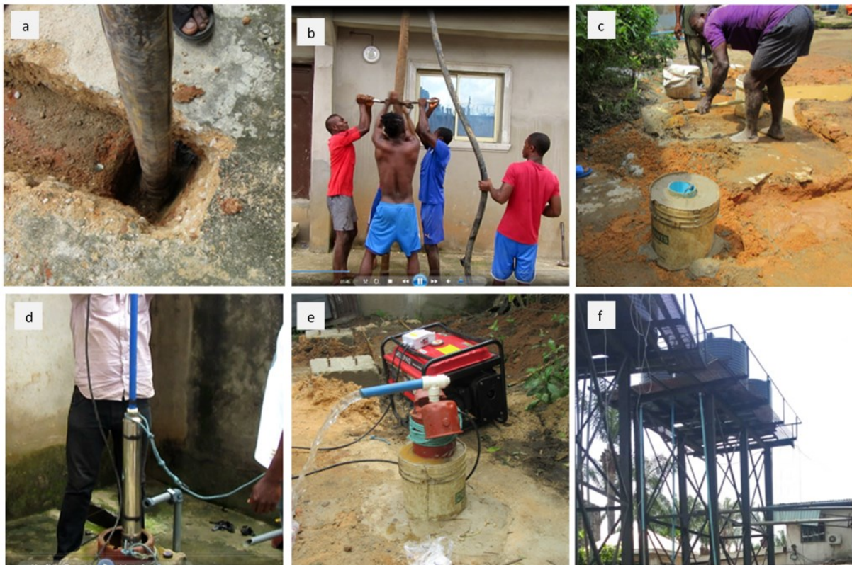
Fig 3-8: Photo Illustration of typical stages in private tube well construction and installation of submersible motor (SUMO) pump in a private resident block in Aba.
