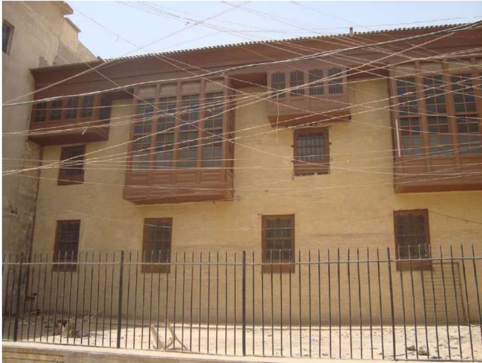
Fig. (4.26): - Jamal Pasha House-Shanashil as decorative element, Source: Photographed by the Author.
