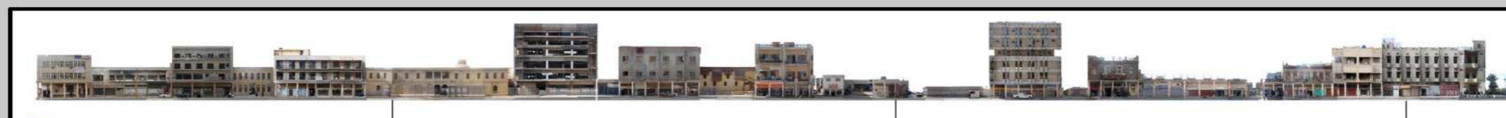
① Traditional and Modern Commercial buildings
