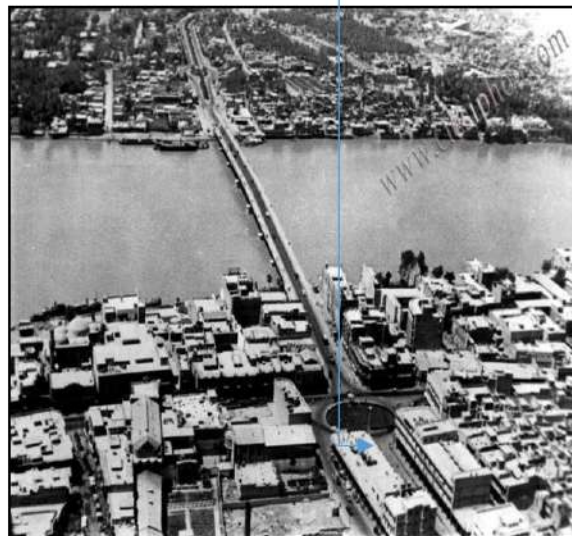
Fig. (4.118): - Hafuth AL-Qathi square and Twin buildings photograph, Source: Iraqi national Archive.
