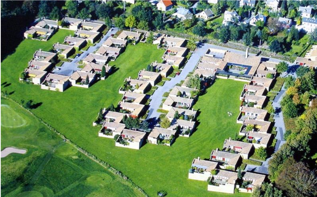
Figure (4.68) View of Fredensborg Housing Source: https://utzon.dk/portfolio-item/fredensborg-housing/
