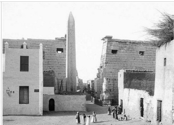
Fig 4.15: Structures in front of Luxor pylon in 1889, to the left is Alsāḥa Alḥajjājia Source: Ali 2011
