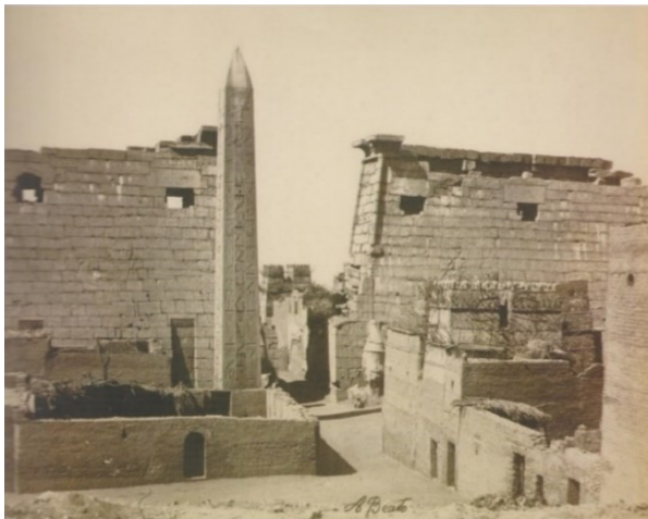
Fig. 4.6: The village and its pigeon towers behind and in front of the pylons of Luxor Temple looking south Source: Ferri 2008
