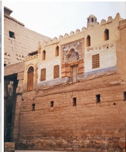
Fig 5.21: Abu Alḥajjāj Mosque from the Ramesside court before restoration Source: Researcher 2004
