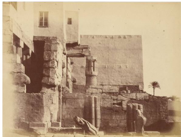
Fig. 4.3: The French House and the ruins of Luxor Temple before 1885 Source: Ali 2011
