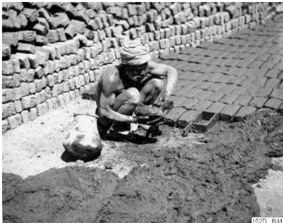
Fig 5.28: Preparing mud bricks in 1924 in Luxor, by Torsten Lenk Source: Lenk N/A
