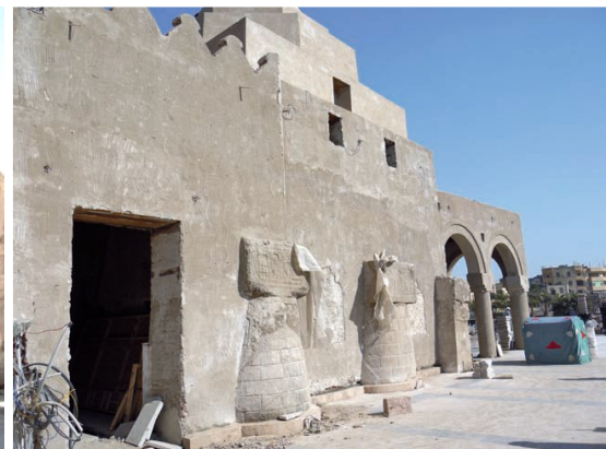
Fig 5.23: Exterior of the restored Abu Alḥajjāj Mosque : the capitals of the Ramesside Portico protruding from the southern wall. Source: Boraik 2008, Pl. XIX
