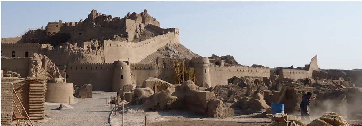
Figure 5-5 View from bazaar to the Governor’s quarter, after the earthquake (Author, 2013)
