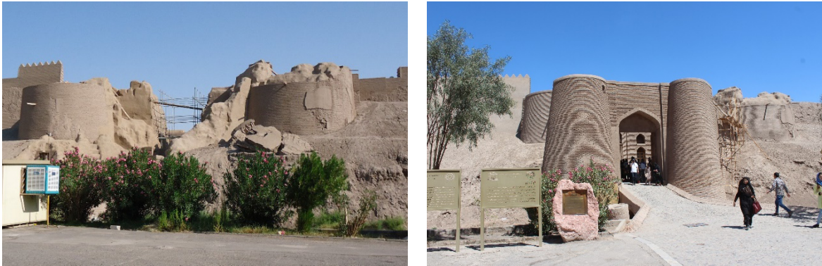
Figure 5-4 left: Main gate after the earthquake (Author, 2013), right: Main gate after the post-earthquake restoration (Sasan Alirezaei, 2018, taken for the author)
