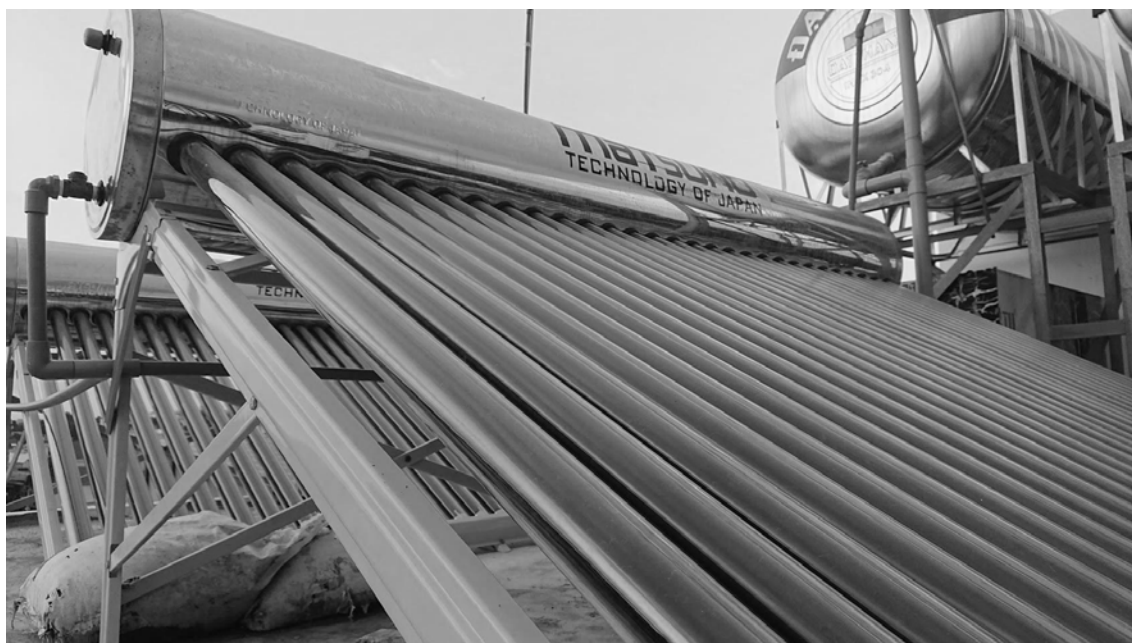
Figure 9–10 Photograph of a typical solar water heating (SWH) system with solar water collectors and storage tank on a rooftop in Da Nang ( source: author's own photograph )
