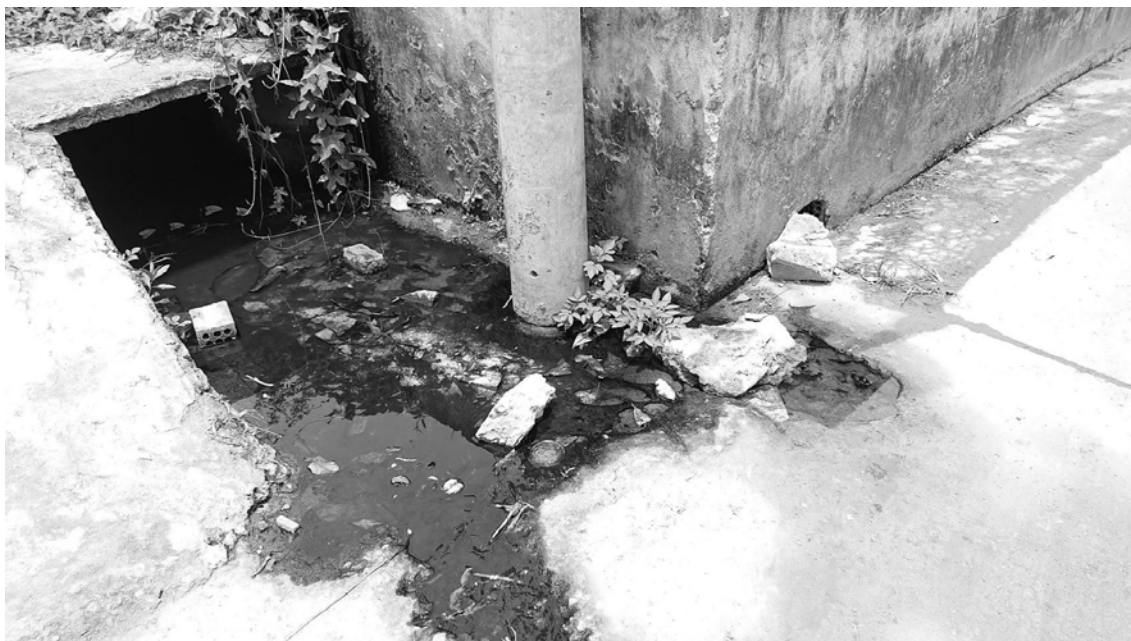
Figure 9–11 Photograph of an open sewer in a peri-urban location (Hòa Khánh Nam/Liên Chiêu District) (source: author's own photograph)
