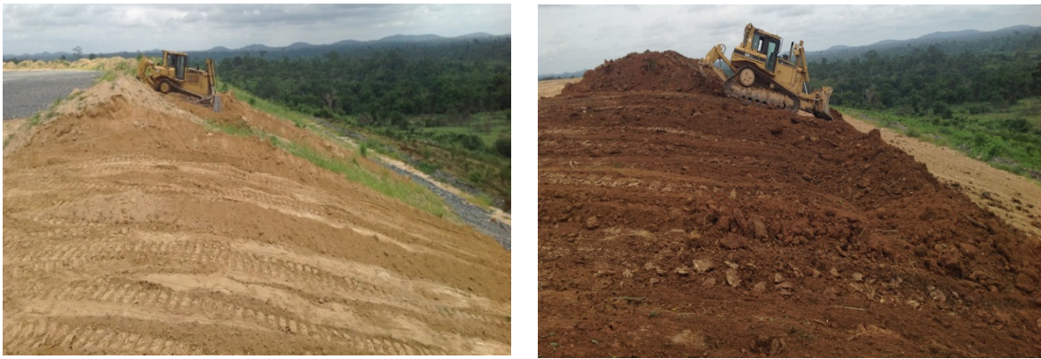
Figure 3. 2: Replacement of stockpiled subsoil (left) and stockpiled topsoil (right).
