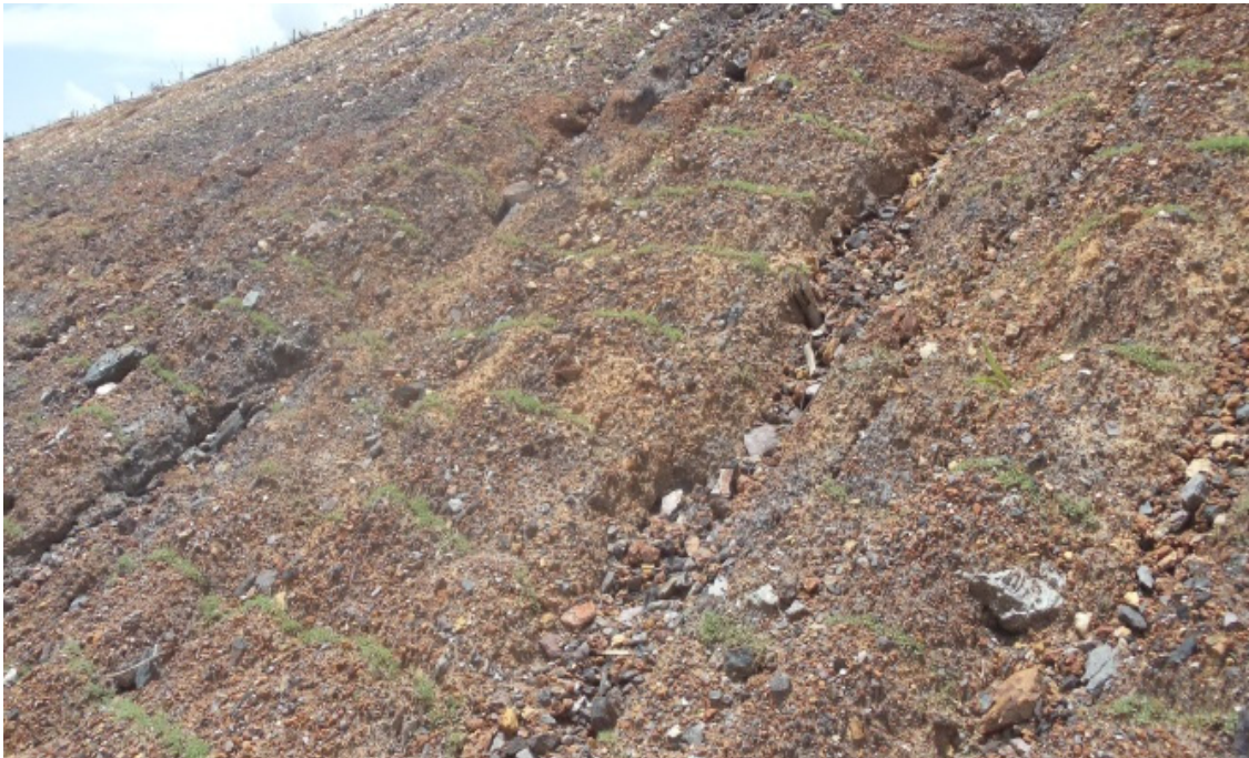
Figure 1. 1: A “reclaimed” mine site in Ghana without slope stabilization, topsoil application or amendment of applied substrate.
