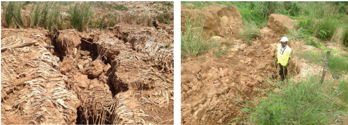
Figure 2. 1: Gully formations following application of the York Mat at NGGL.
