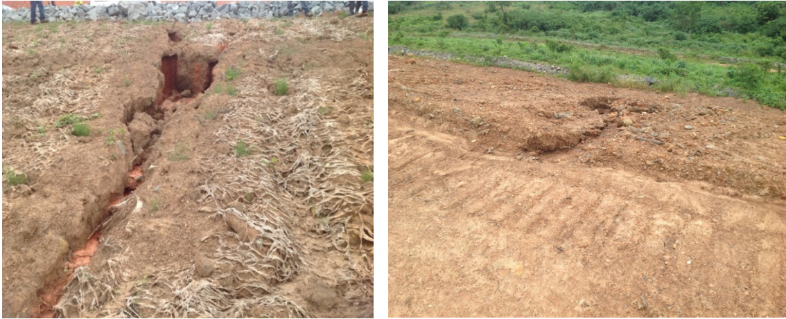
Figure 2. 11: Gully formations during reclamation at NGGL.
