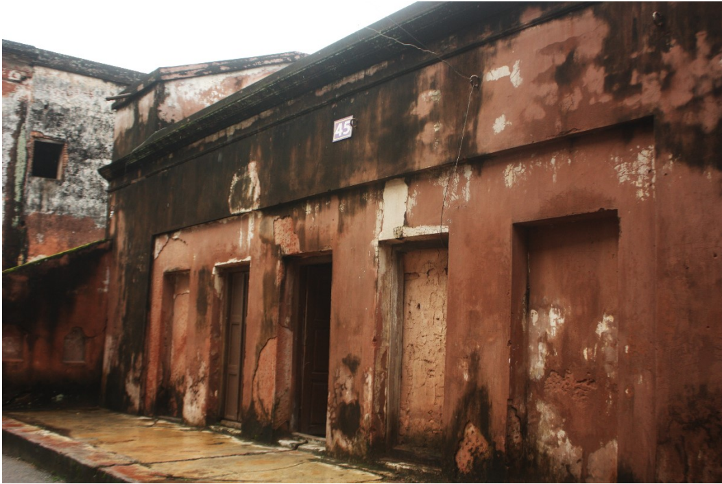
Figure 12: Compartment type building Source: Author
