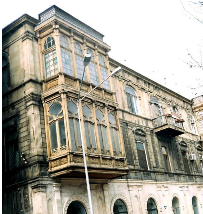
Figure 4: Shushebend of a residential building at 4 A. Zeynalli
