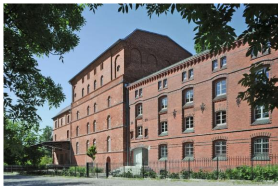
Figure 2: Fuerstenwalde mill after renovation in Brandenburg
