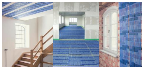
Figure 1: The application of capillary mats in rooms
