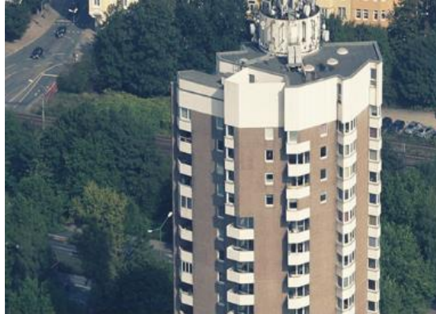
Figure 4: Apartment house in Osnabruck
