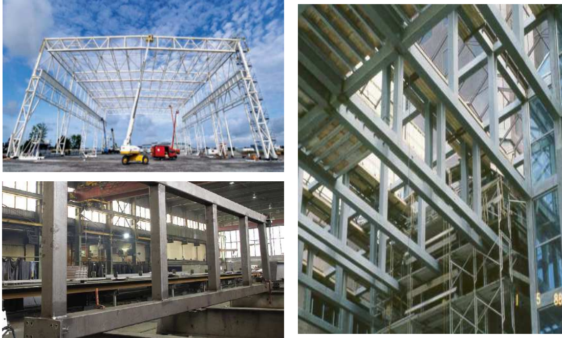
Figure 2.1: Application of SHS T-joints in buildings [24] and [25].
