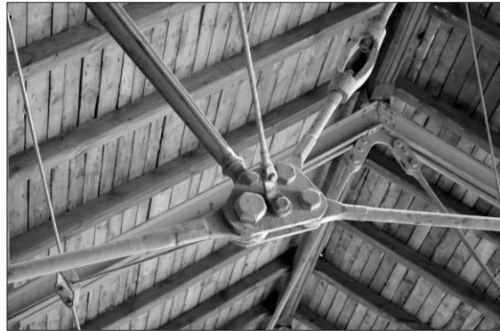
(c) Similar form of the Wiegmann–Polonceau truss to the one at Reithalle Potsdam
