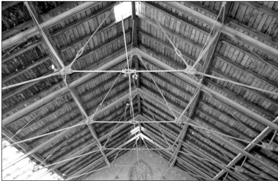
(c) Similar form of the Wiegmann–Polonceau truss to the one at Reithalle Potsdam
